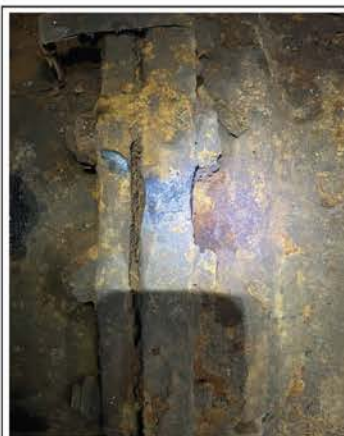
CO Vault 3 - Flange
