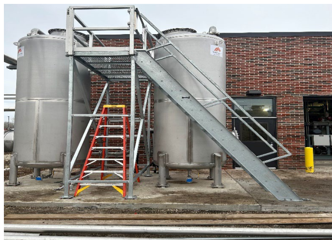
Siloxane Removal Tank Stair Installation
