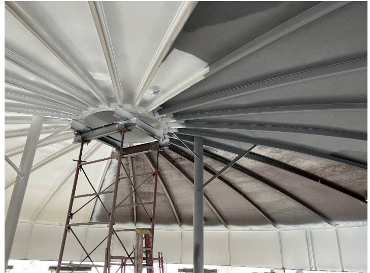
Digester 3 Cover Coating Process
