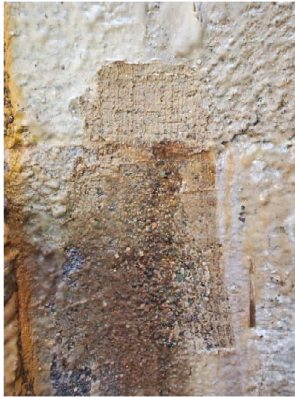
Photo 13 – MH 89 Wall Condition – Growth Removed
