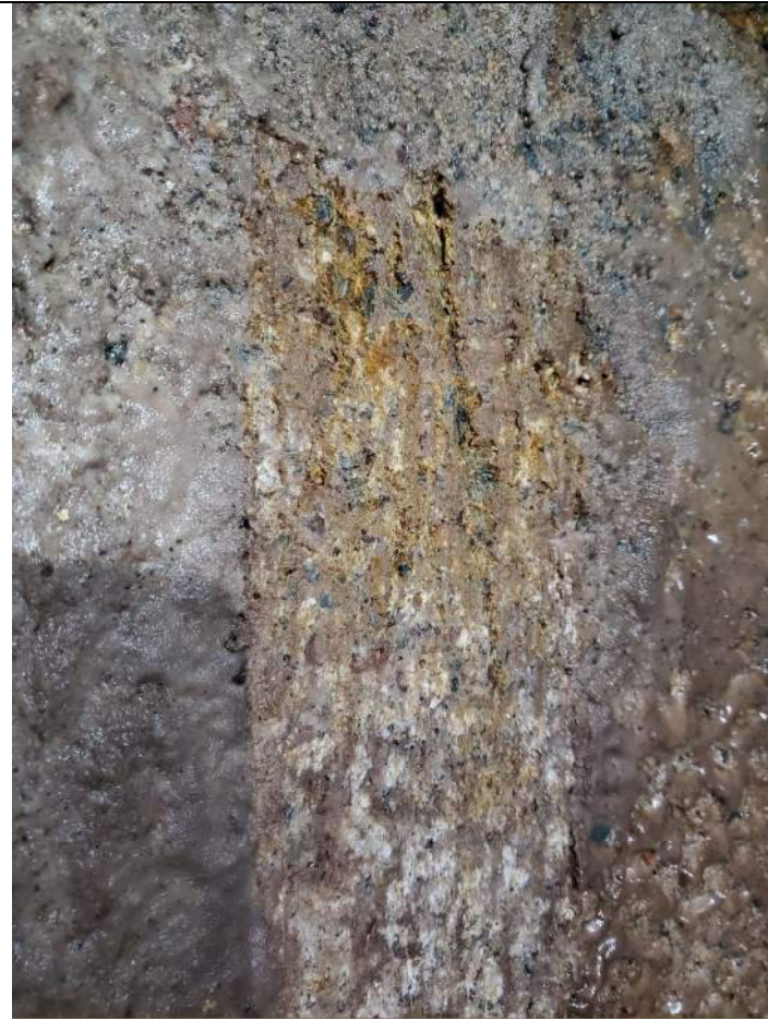
Photo 5: Compitent Concrete MH wall after film scraped away
