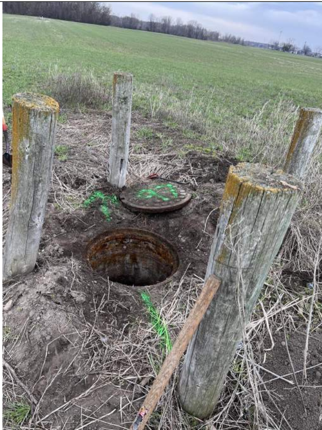
Photo 1: MH 97 Rim and Casting
