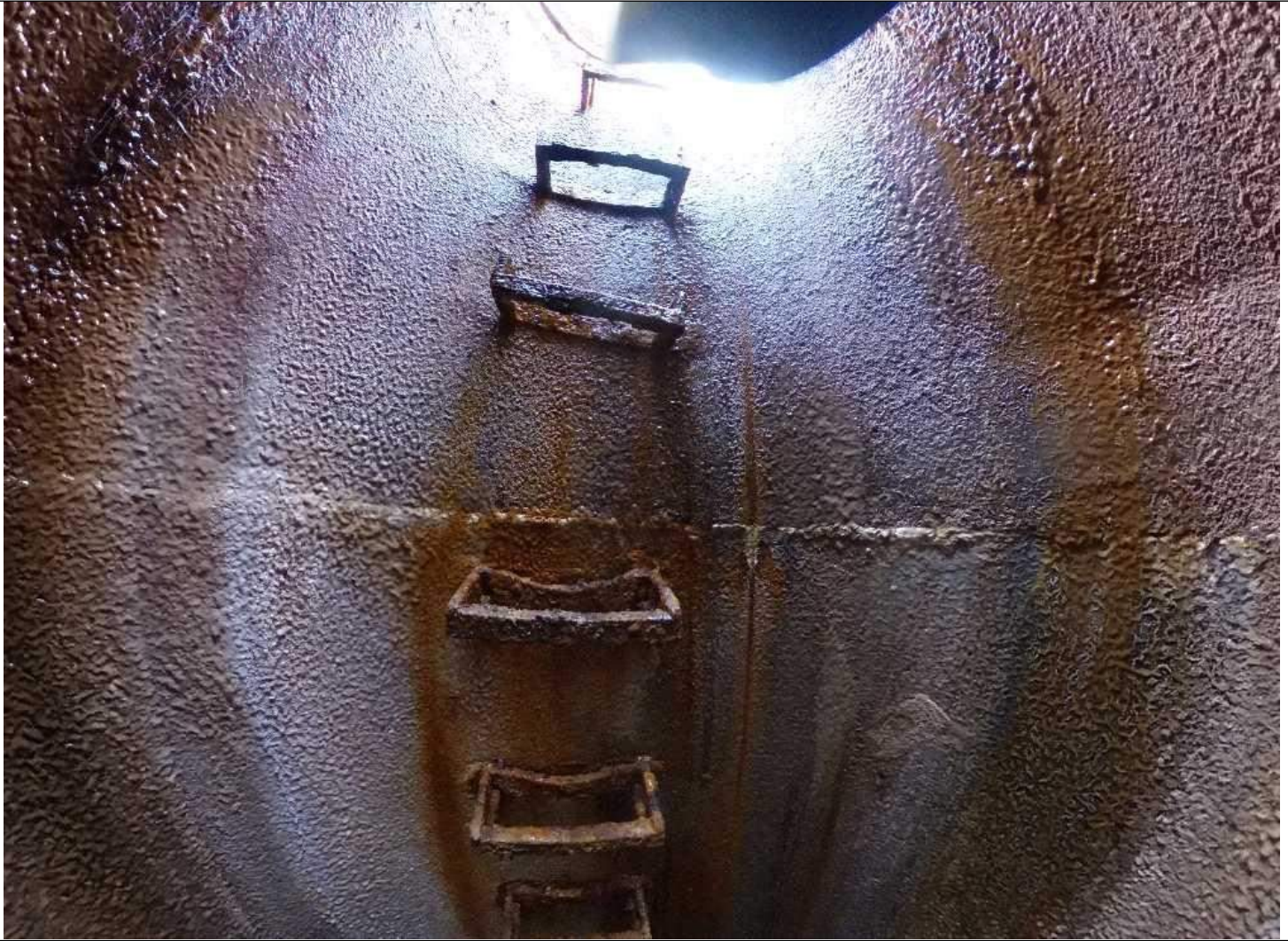
Photo 5: MH 78 Image Capture from 360° Camera, Showing stained, wet and milky like substance on walls
