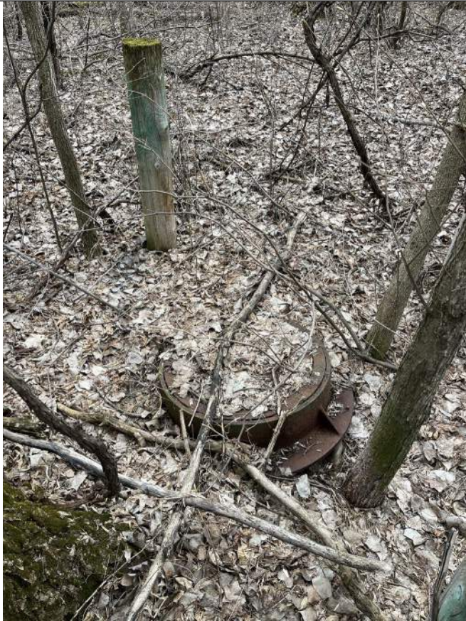
Photo 1: MH 95 Rim and Casting
