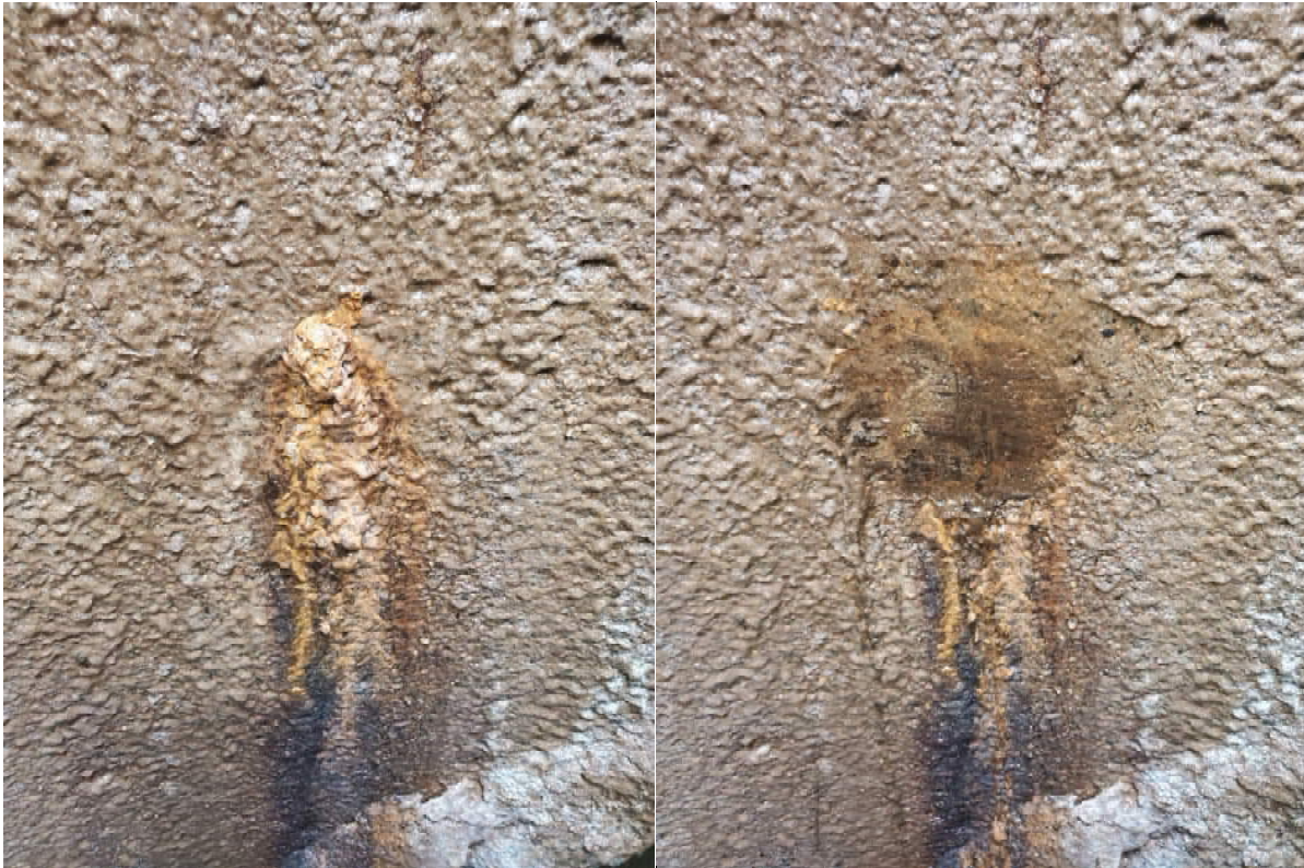
Photo 23 – MH 98 Infiltration Buildup
