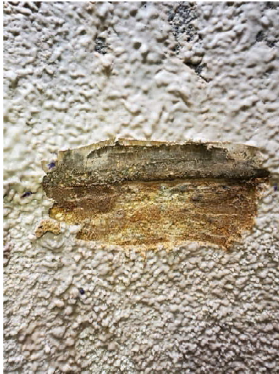
Photo 8 – MH 80 Wall Condition at Riser Joint – Growth Removed
