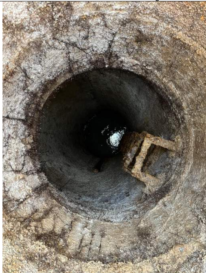
Photo 3: MH 93 Roots on Cone Section
