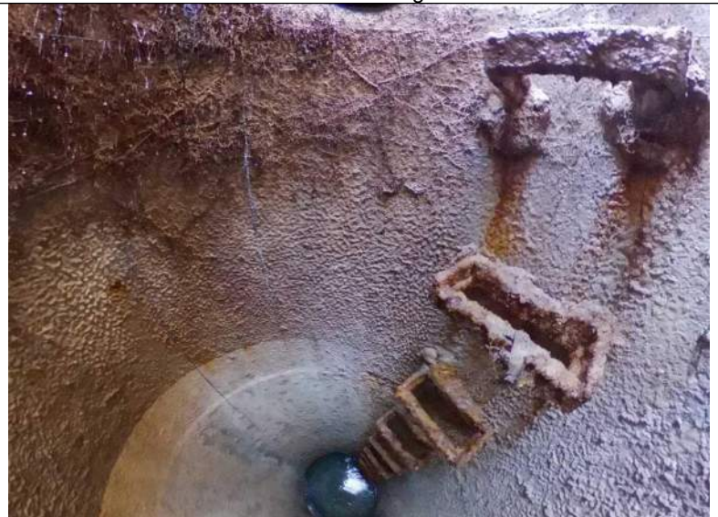
Photo 2: MH 93 Casting and Cone
