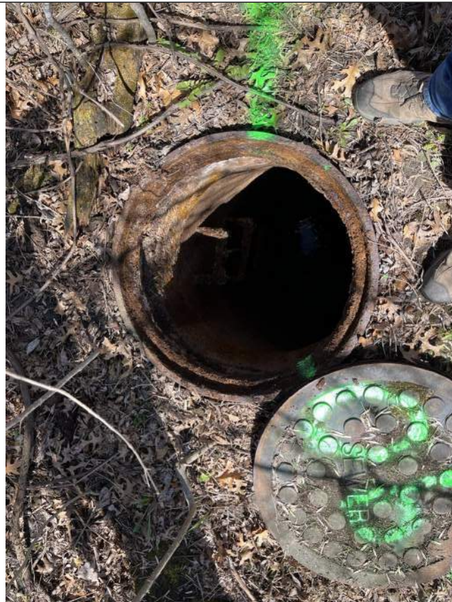
Photo 2: MH 90 Rim and Casting
