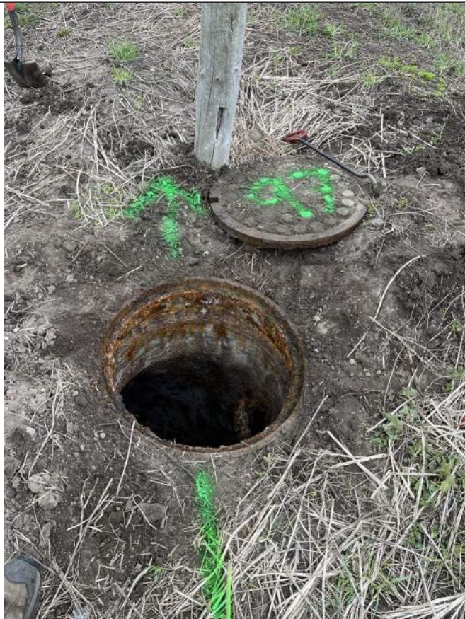
Photo 2: MH 97 Rings and Cone
