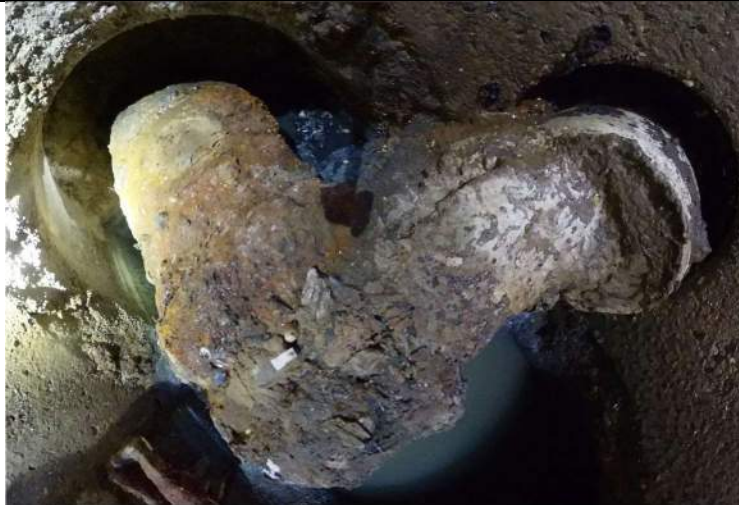
Photo 3: MH 113 Force main (Left) Bulkhead (Right) top view.
