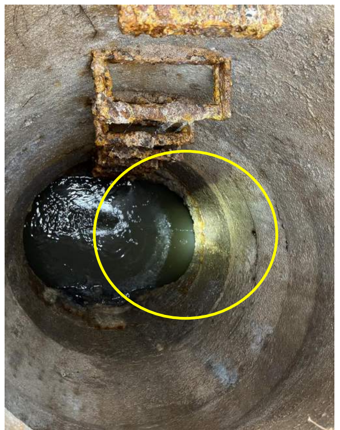
Photo 4: MH 96 Light on the leaking joint
