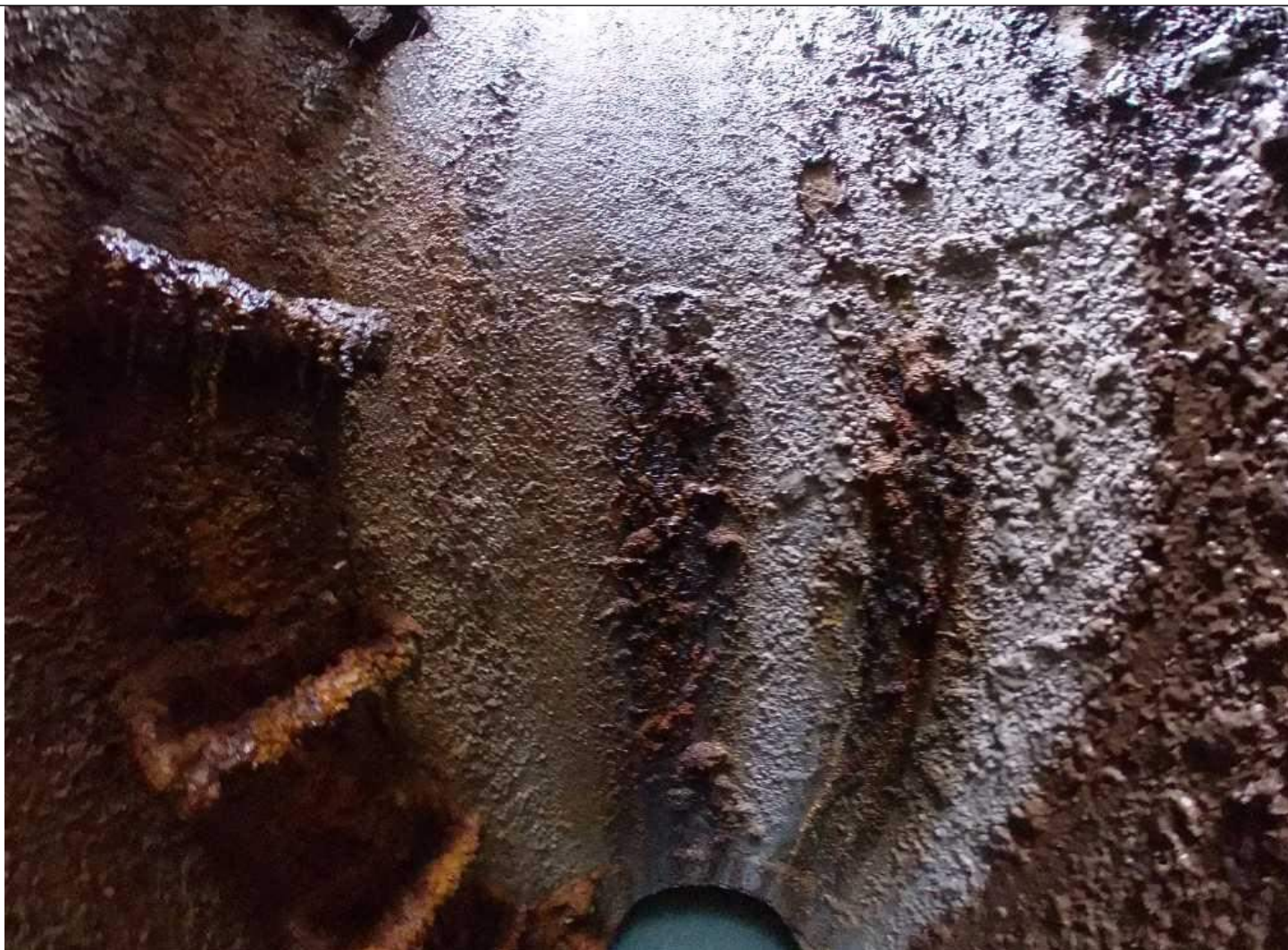
Photo 5: MH 81 Image Capture from 360° Camera, Showing stained, wet walls.
