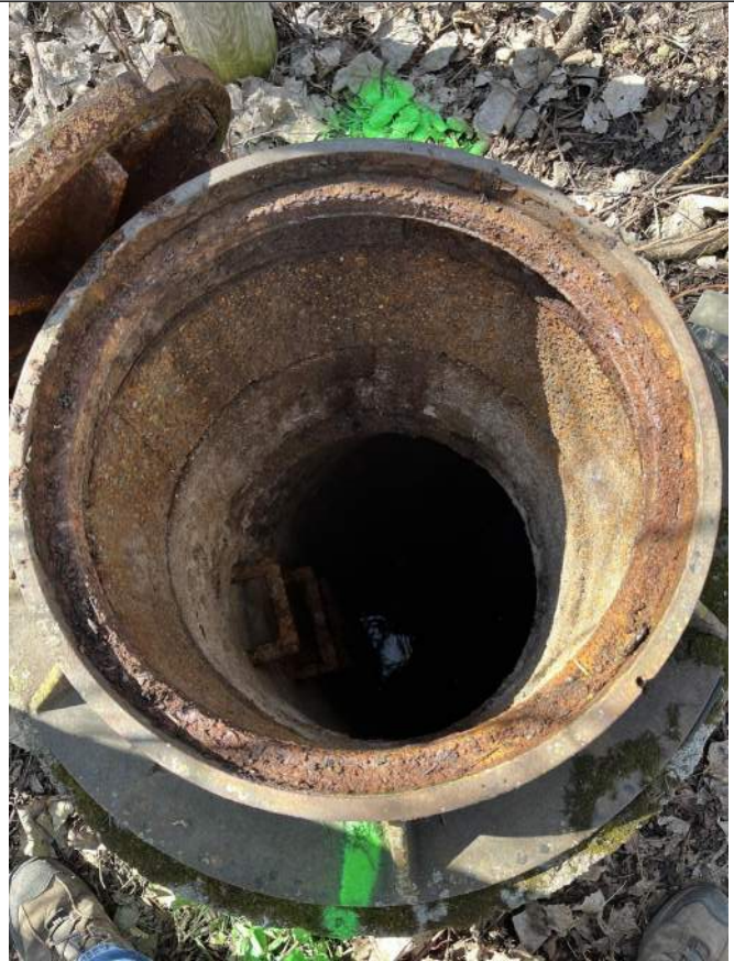
Photo 2: MH 92 Casting, Riser, and Cone
