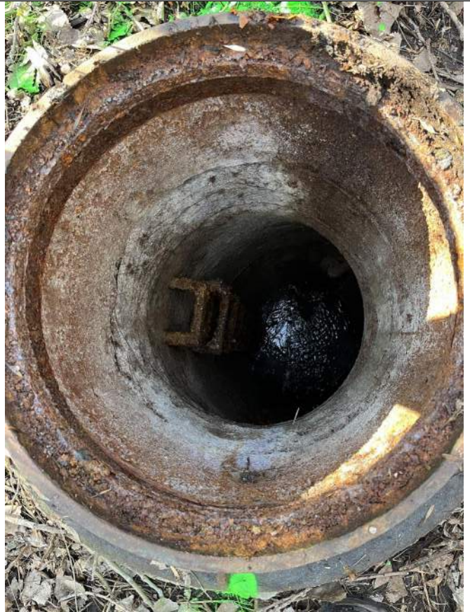
Photo 2: MH 94 Casting and Cone
