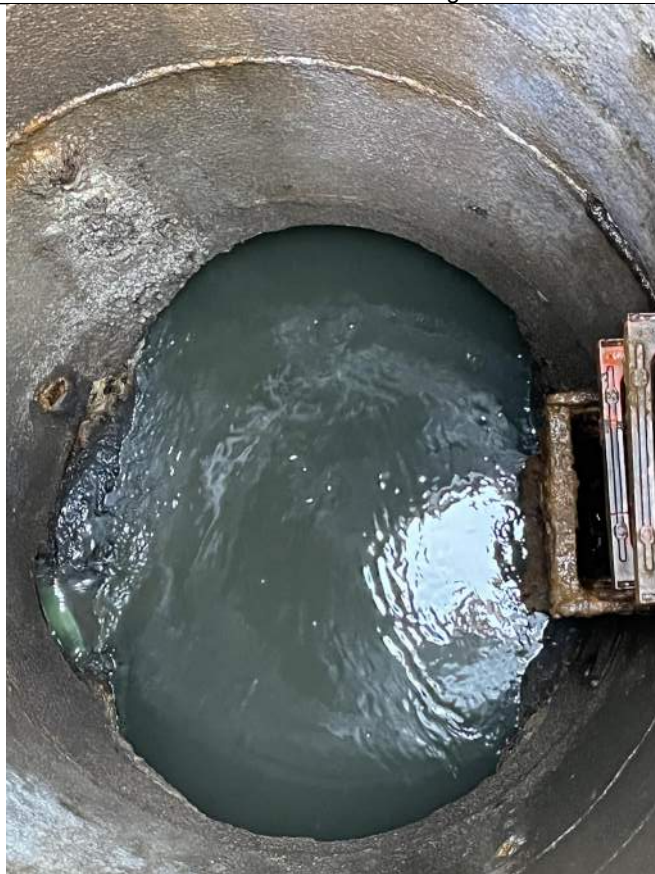
Photo 4: MH 99, 10" PVC inlet at lower left
