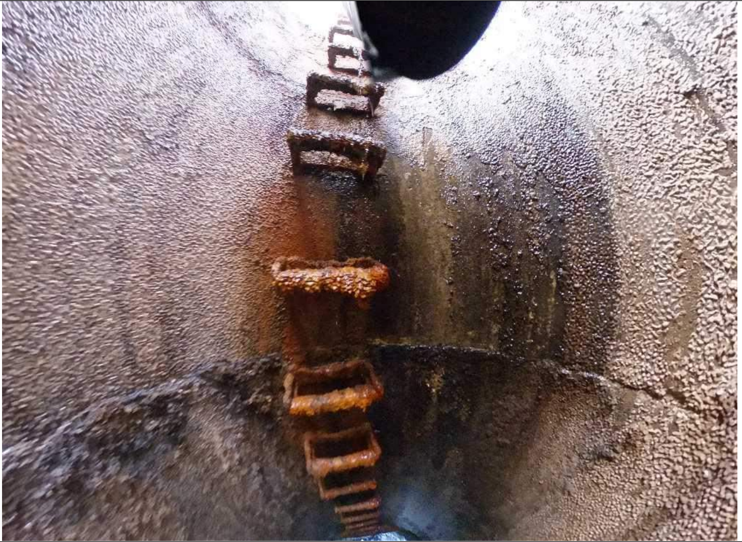
Photo 5: MH 84 Image Capture from 360° Camera, Showing stained walls and weeping walls
