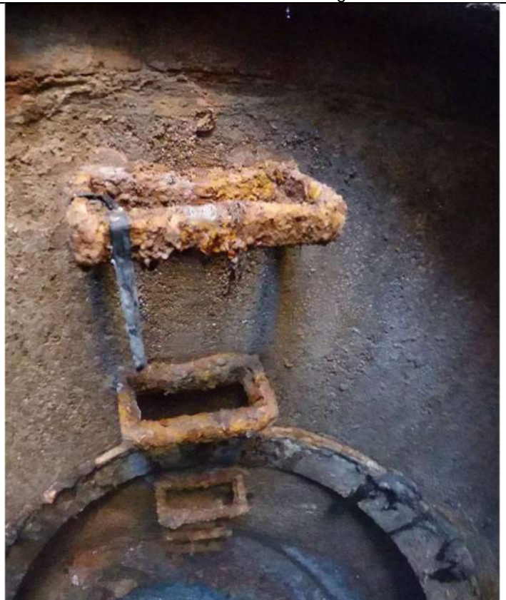
Photo 4: MH 102 Stairs Brick layer on top section of barrel are less competent than barrel section, but in fair condition.
