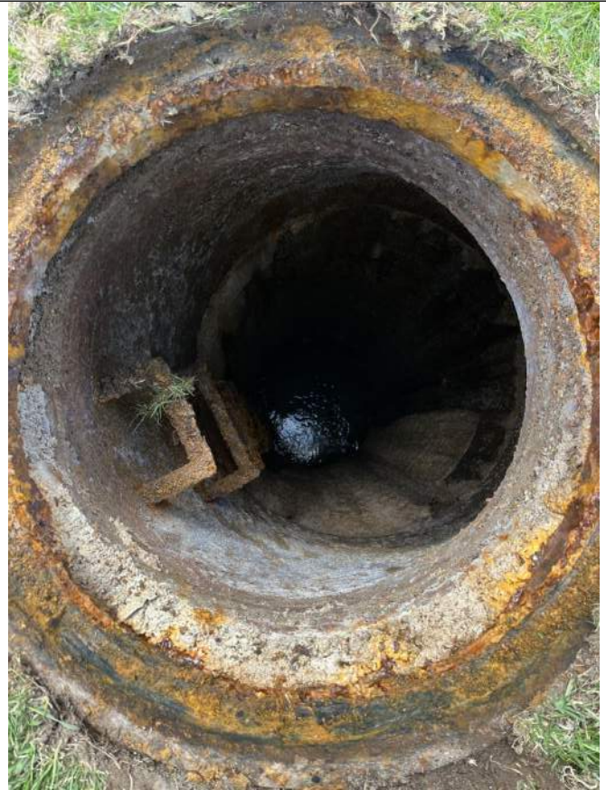
Photo 2: MH 91 Casting, and Cone
