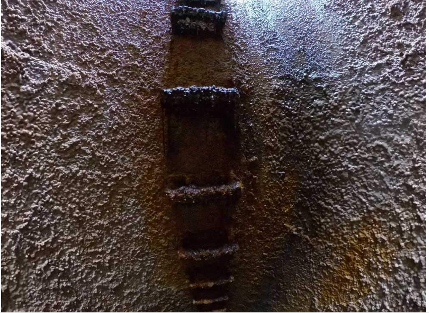
Photo 5: MH 80 Image Capture from 360° Camera, Showing stained, weathered concrete
