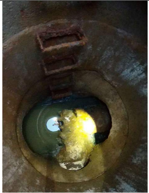
Photo 2: MH 113 Ladder and pipes
