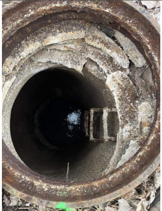
Photo 2: MH 95 Broken Rings and Cone
