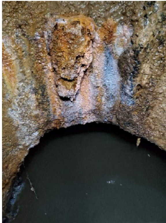
Photo 18 – MH 92 Wall Condition at Interceptor Pipe
