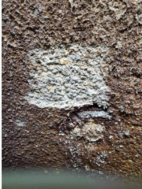
Photo 1 – MH 78 Cone Section Wall Condition – Growth Removed
