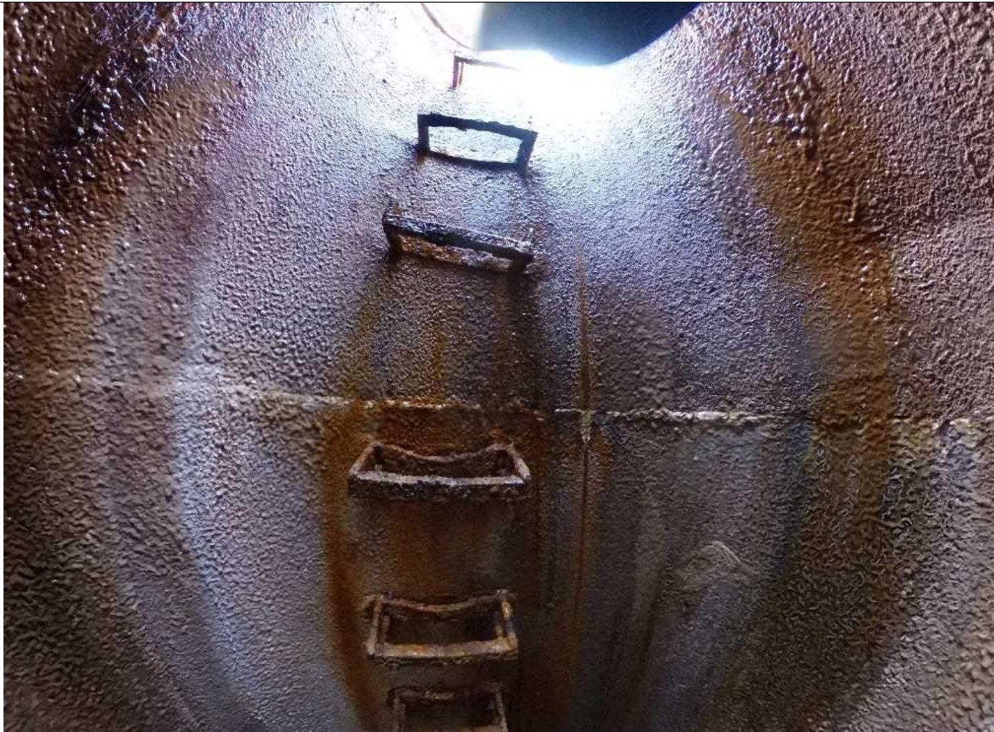
Photo 5: MH 79 Image Capture from 360° Camera, Showing stained, milky like substance on walls
