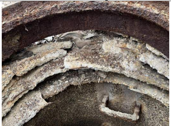
Photo 2: MH 95 Broken Rings and Cone
