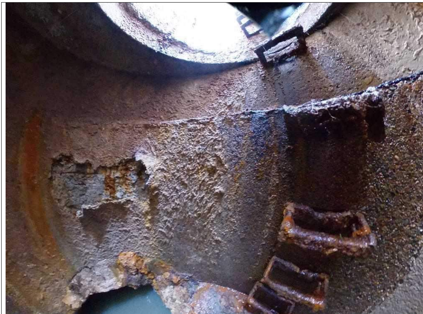
Photo 4: MH 89 Image Capture from 360° Camera, Showing inlet pipe, concrete spalling and stained walls
