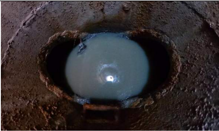
Photo 3: MH 111 Debris caught on edge of pipe
