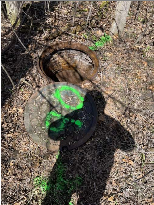
Photo 1: MH 90 Rim and Casting
