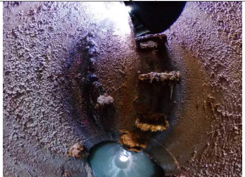
Photo 2: MH 92 Casting, Riser, and Cone
