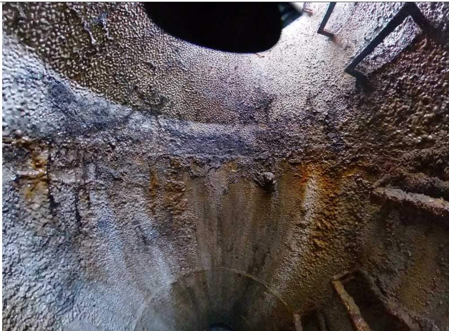
Photo 5: MH 85 Image Capture from 360° Camera, Showing stained walls
