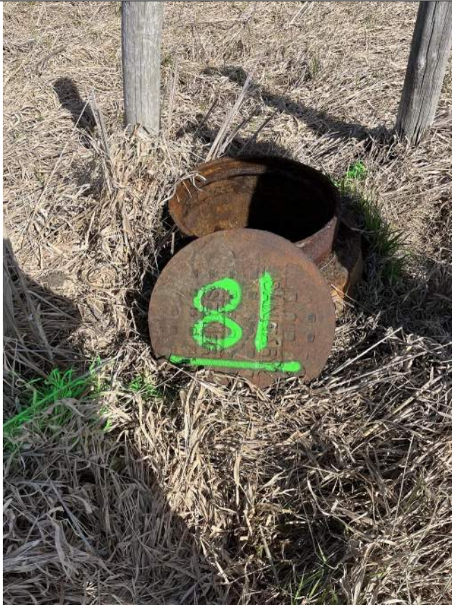
Photo 1: MH 81 Cover and Casting
