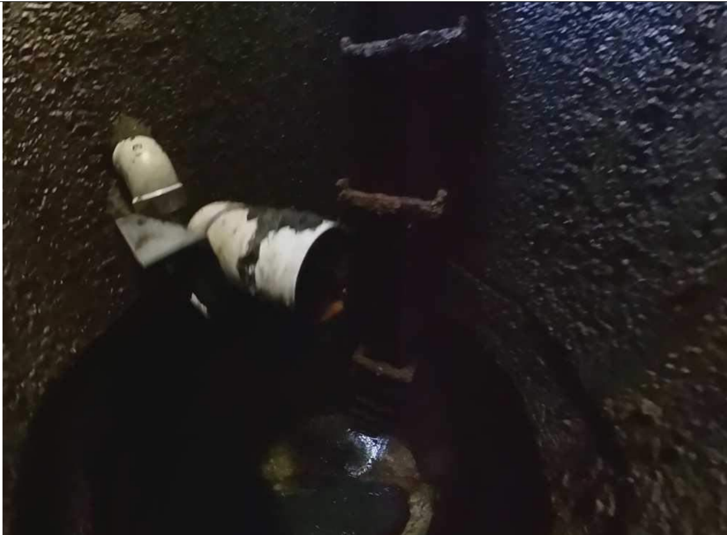
Photo 5: MH 77A Image Capture from 360° Camera, showing unknown PVC pipe with a trap
