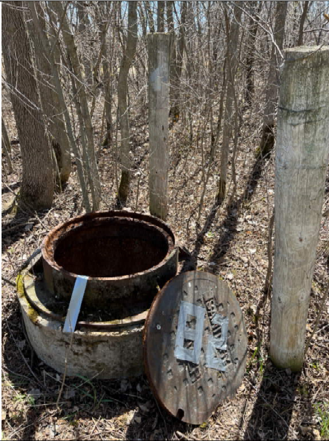
Photo 1: MH 82 Cover and Casting
