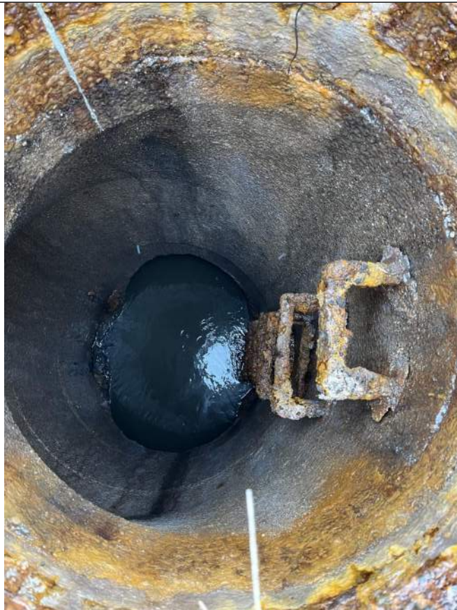
Photo 2: MH 98 Rings and Cone
