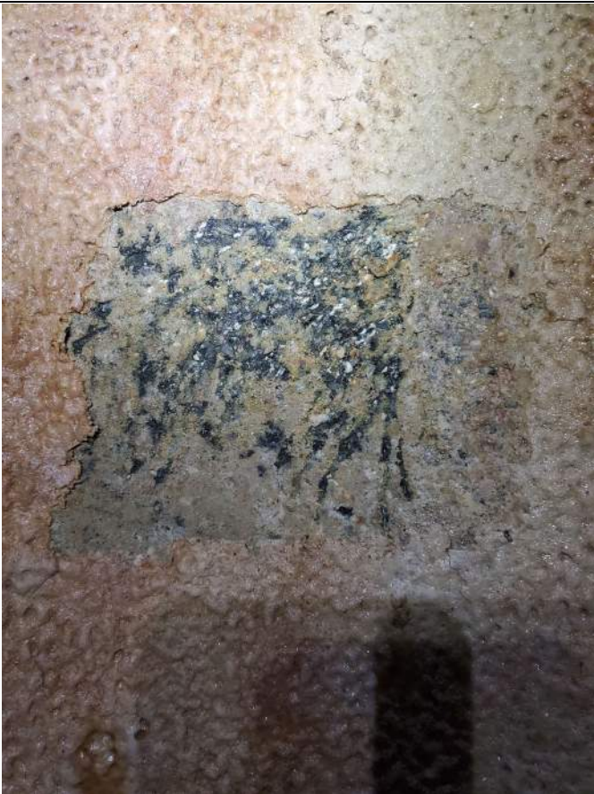
Photo 3: Slime and black coating on MH walls
