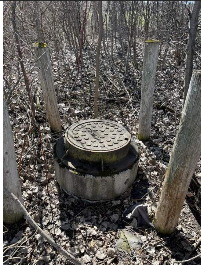
Photo 1: MH 92 Riser, Rim, and Casting
