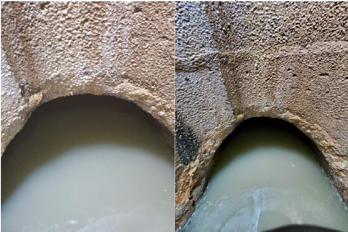
Photo 24 – MH 98 Wall Condition at Interceptor Pipe
