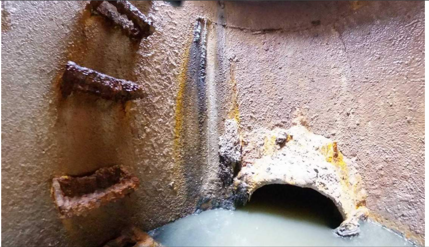
Photo 4: MH 89A Image Capture from 360° Camera, Showing inlet pipe and stained walls
