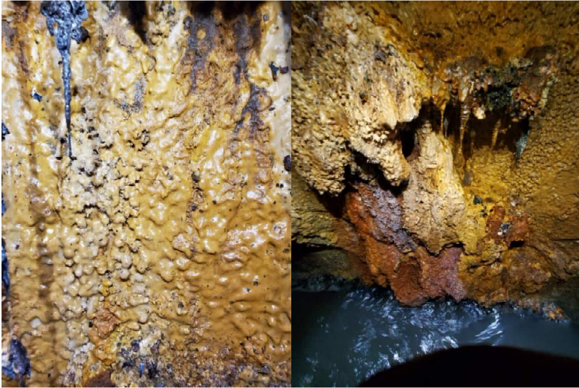
Photo 9 – MH 80 Mineral Buildup
