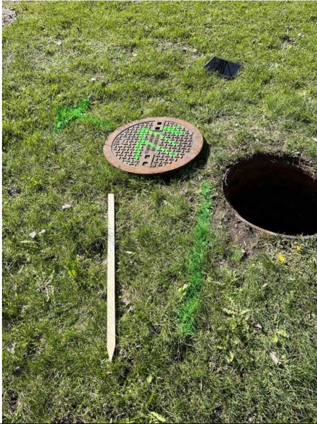
Photo 1: MH 77A Cover and Casting
