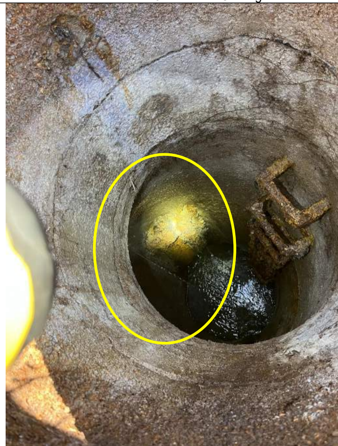
Photo 3: MH 94 Leaking Joint and buildup on wall
