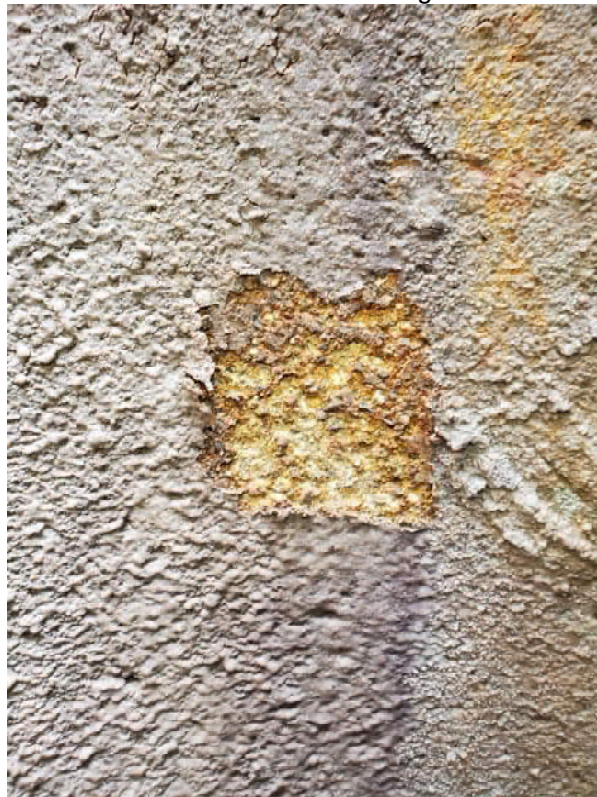
Photo 4 – MH 80 Top Riser Section Wall Condition – Growth Removed
