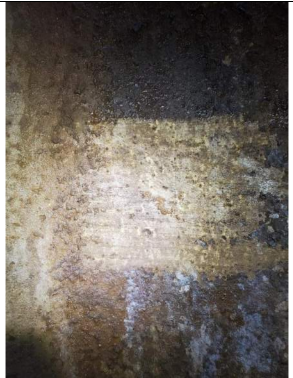
Photo 4: MH 111 Worm holes in concrete wall, but competent concrete
