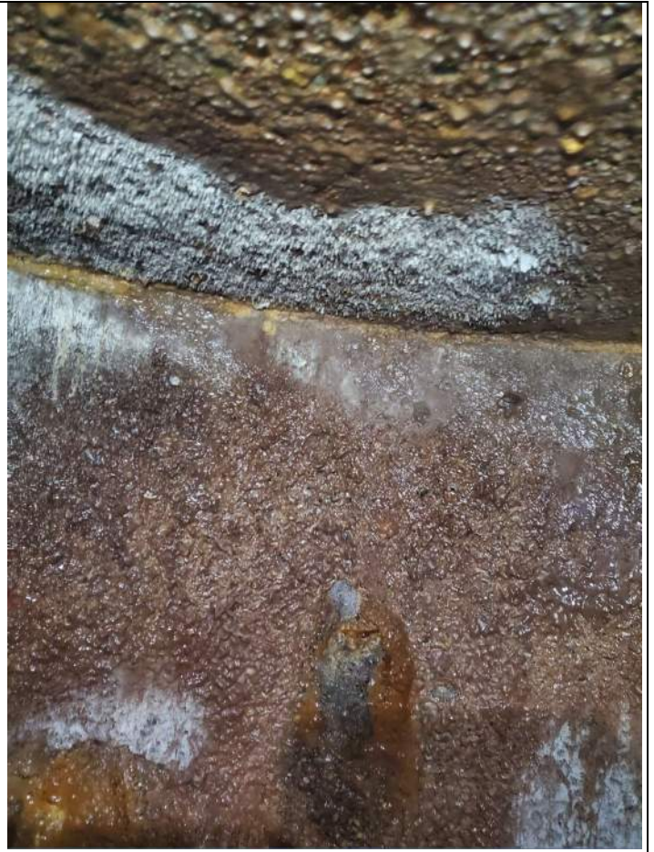
Photo 6: Compitent concrete flat top sitting on 6' bottom section
