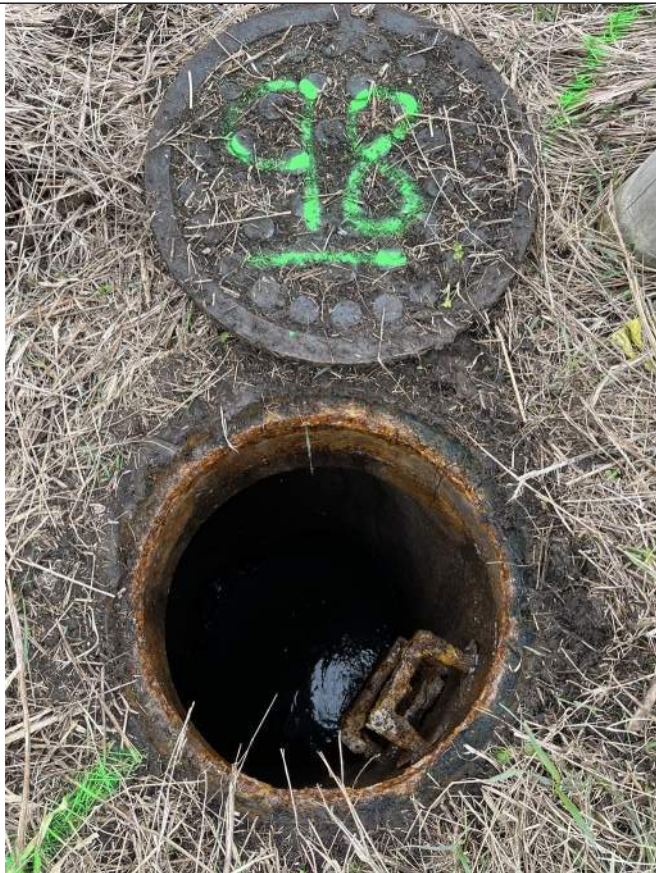
Photo 1: MH 98 Rim and Casting
