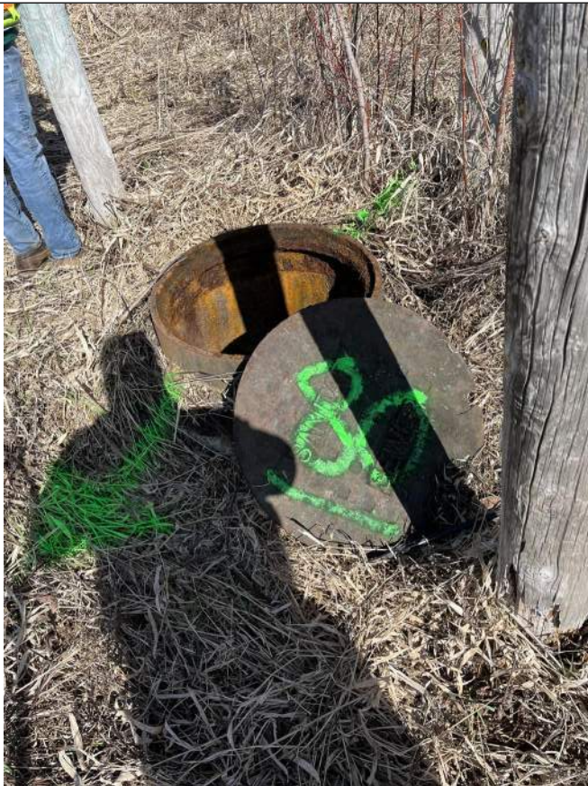
Photo 1: MH 80 Cover and Casting
