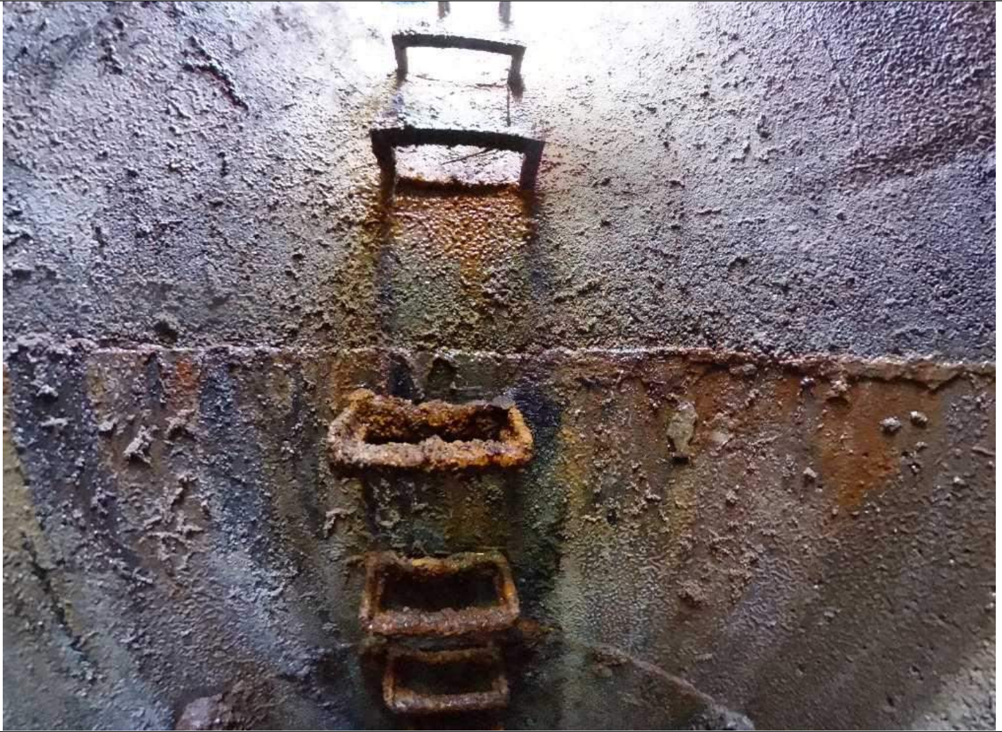
Photo 5: MH 86 Image Capture from 360° Camera, Showing stained walls and dripping coming the steps
