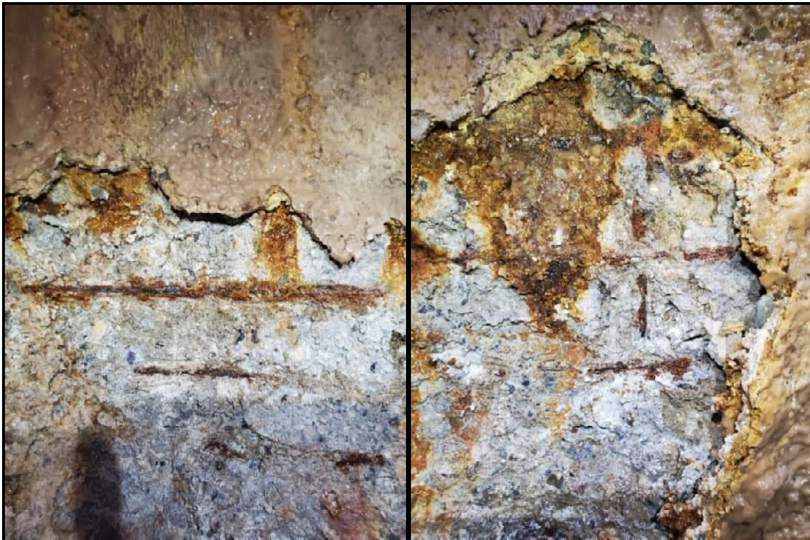
Photo 14 – MH 89 Wall Condition - Exposed Rebar
