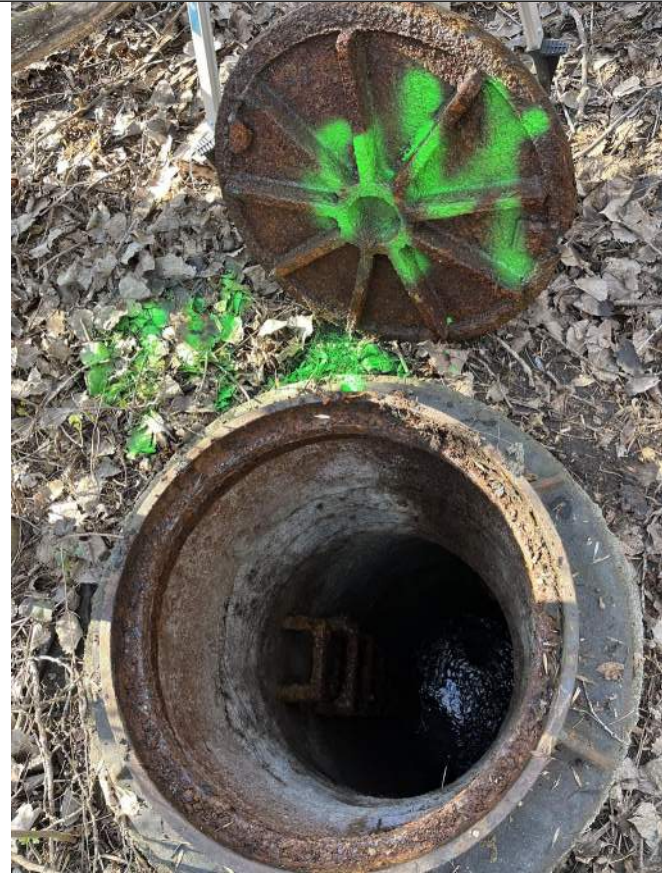
Photo 1: MH 94 Rim and Casting
