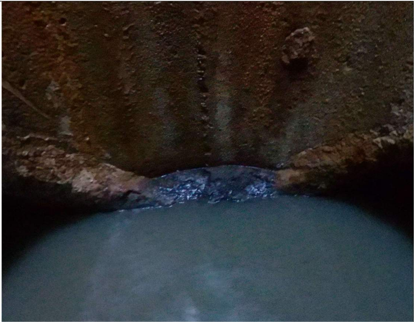
Picture 4: Eroded Remains of Bench
