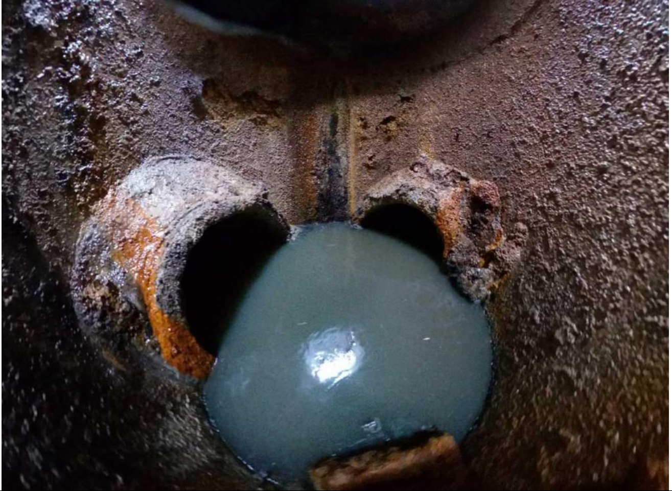
Photo 4: MH 90 Image Capture from 360° Camera, Showing inlet pipe on left and outlet pipe on right
