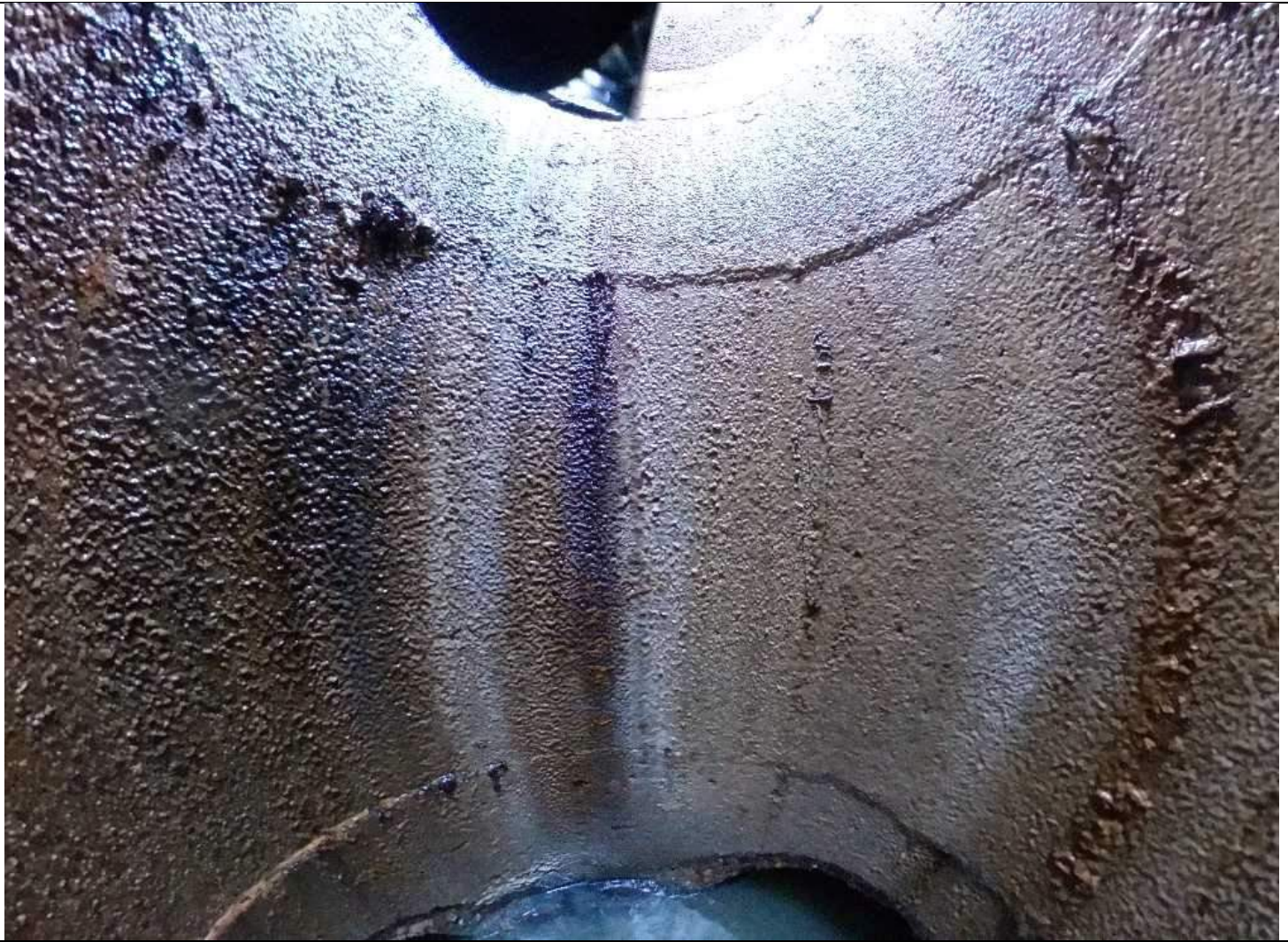
Photo 5: MH 87 Image Capture from 360° Camera, Showing stained walls
