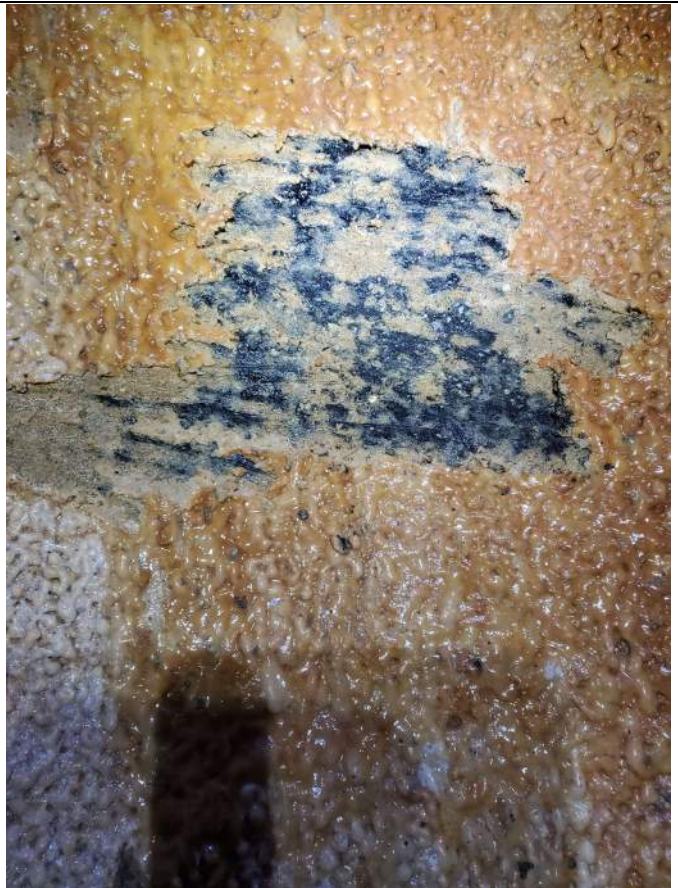
Photo 4: Slime and black coating on MH walls
