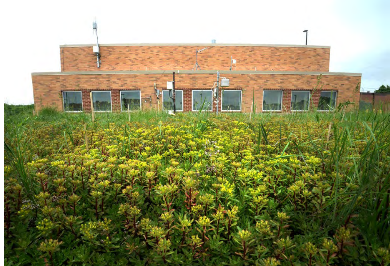
Image of Green Roof at the MCES Empire Wastewater Treatment Plant in Farmington, MN
