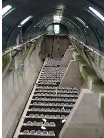
Figure 5. Aeration Tank Diffusers.
