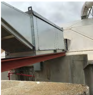
Figure 7. Primary Clarifier Make-Up Air Unit.
