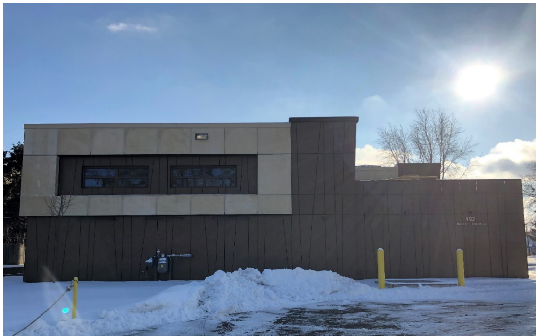
Lift station facing Hiawatha Avenue in Hopkins
