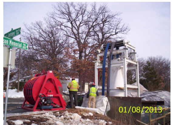
Example of CIPP inversion process.
