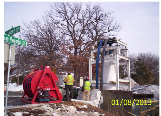
Example of CIPP inversion process.
