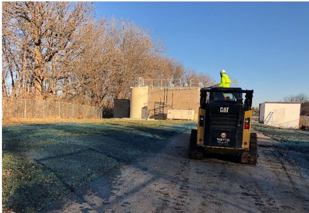
Crews are hydroseeding the land at the lift station and at the property adjacent to the lift station in preparation for winter.
