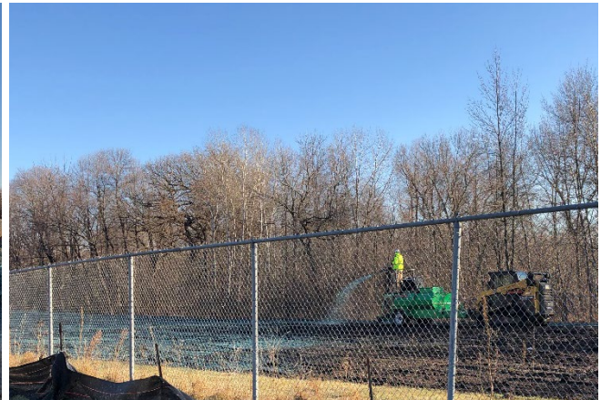
Crews are hydroseeding the land at the lift station and at the property adjacent to the lift station in preparation for winter.
