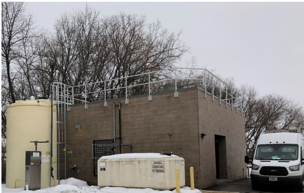
Crews arrive to work on the interior of the lift station in Maple Plain
