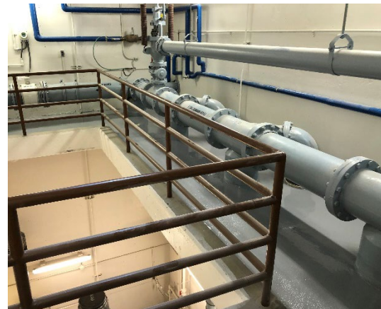
Top + Bottom Picture: Freshly coated floors inside the lift station
