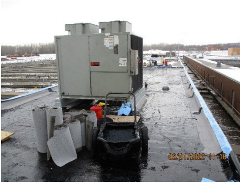
ESE2 Built-Up Roof Construction
