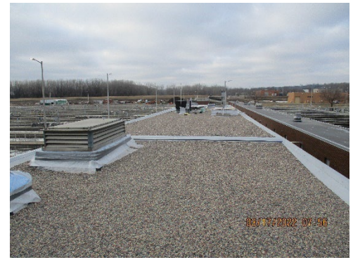
ESE2 Roof Construction Complete
