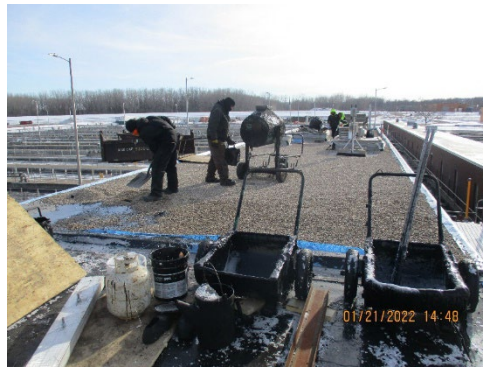
ESE2 Built-Up Roof Construction
