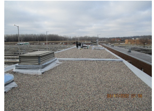
ESE2 Roof Construction Complete
