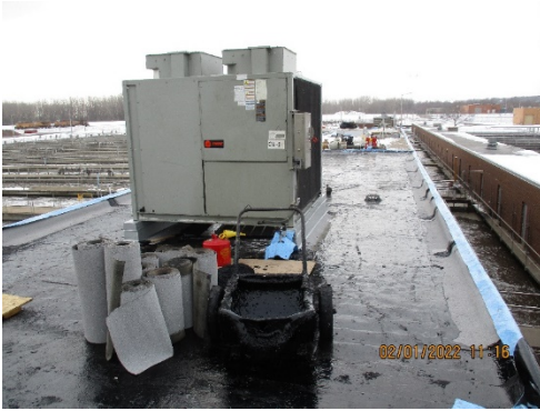
ESE2 Built-Up Roof Construction
