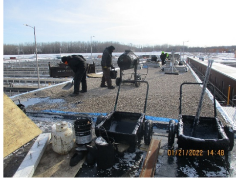
ESE2 Built-Up Roof Construction
