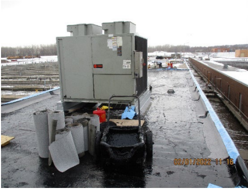
ESE2 Built-Up Roof Construction
