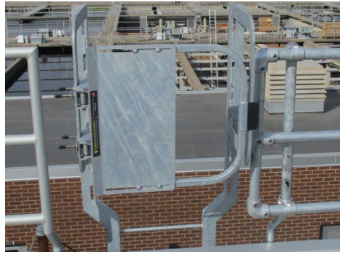
New Ladder on ESE2 Roof
