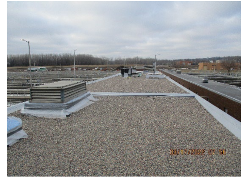
ESE2 Roof Construction Complete
