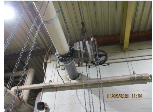
New BF08 Vent Piping at the 408 Building
