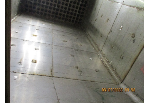
Baghouse No. 1 New Stainless Steel Liner
