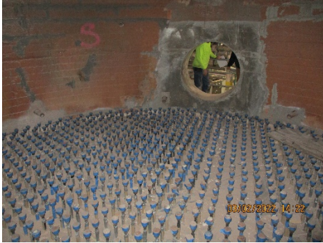
Incinerator No. 1 New Tuyeres Installed Before Pouring Refractory
