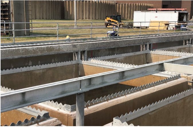
Concrete Work at PST 8
