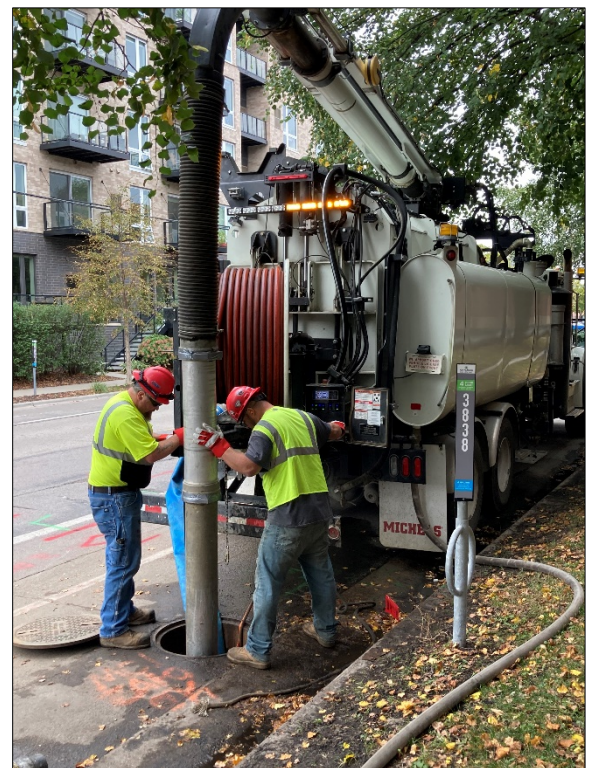
Crews cleaning a section of the sanitary sewer
