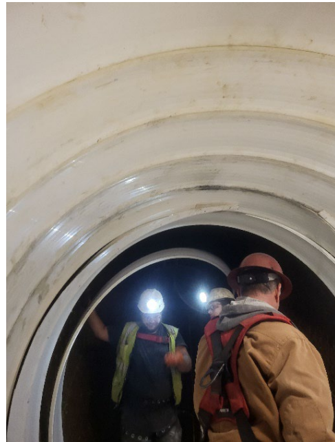
Crew members install liner under Marshall Street.
