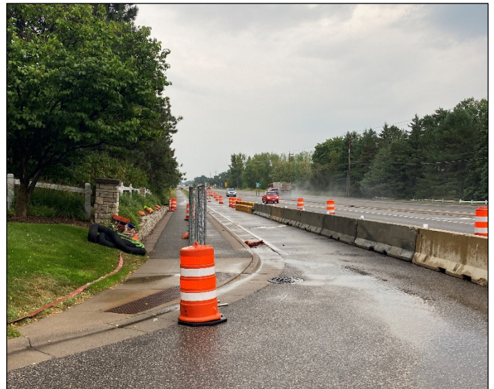
Barrier installation before excavation near Lake Drive and Antrim Road
