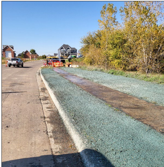
Crews completing soft surface restoration
