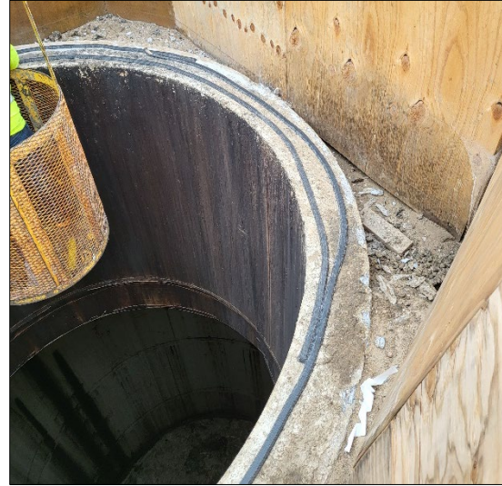
Crews preparing to cover access pipe
