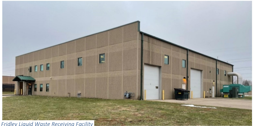
Fridley Liquid Waste Receiving Facility
