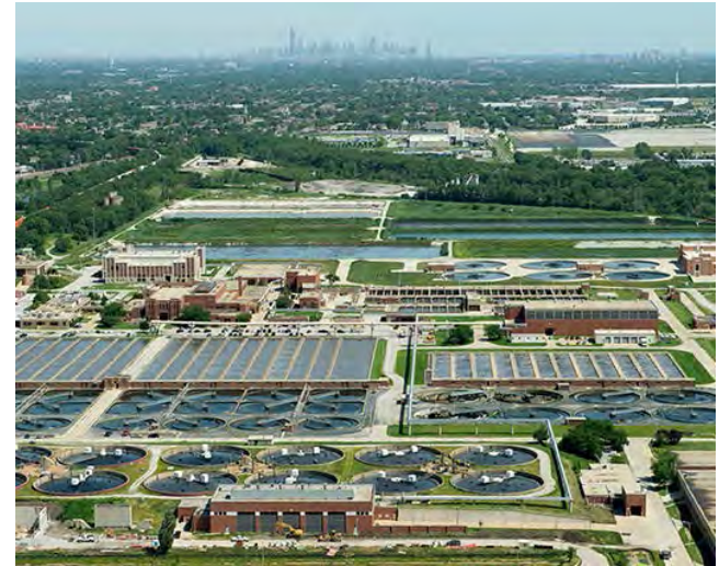
Calumet Water Reclamation Plant
