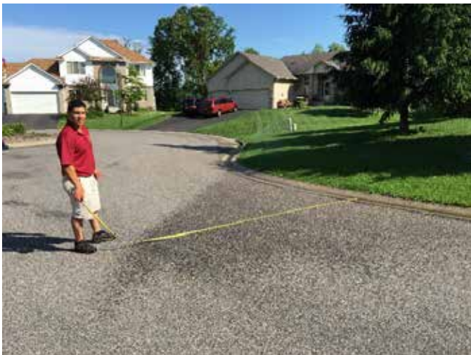
Figure 28: Wet road surface due to improperly adjusted rotor head
