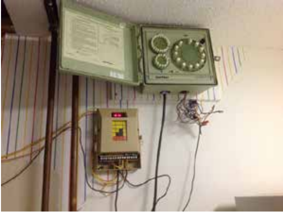
Figure 37: Dated irrigation technology (Rainbird RC 1260)
