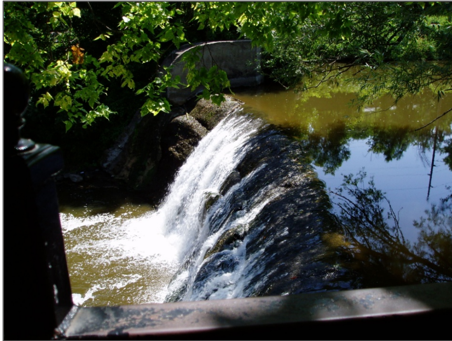
Figure SA-3: Dam on Sand Creek immediately upstream of Jordan, Minnesota
