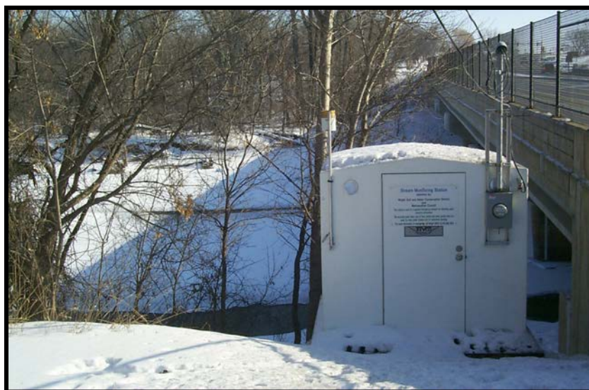
Figure CW-1: Crow River Station below Highway 55 near Rockford (CW 23.1)
