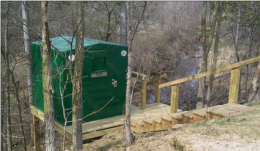
Figure BR-1: Browns Creek at Dellwood Road
