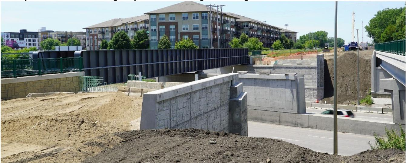
Crews have almost completed the pier and abutments needed in this area and are working on finishing details. Construction of freight rail infrastructure in the area is also underway. When complete, the freight rail bridge, pictured on the left, will be picked up and moved onto the newly constructed bridge foundation. The LRT bridge will be built where the freight rail bridge is currently located.
