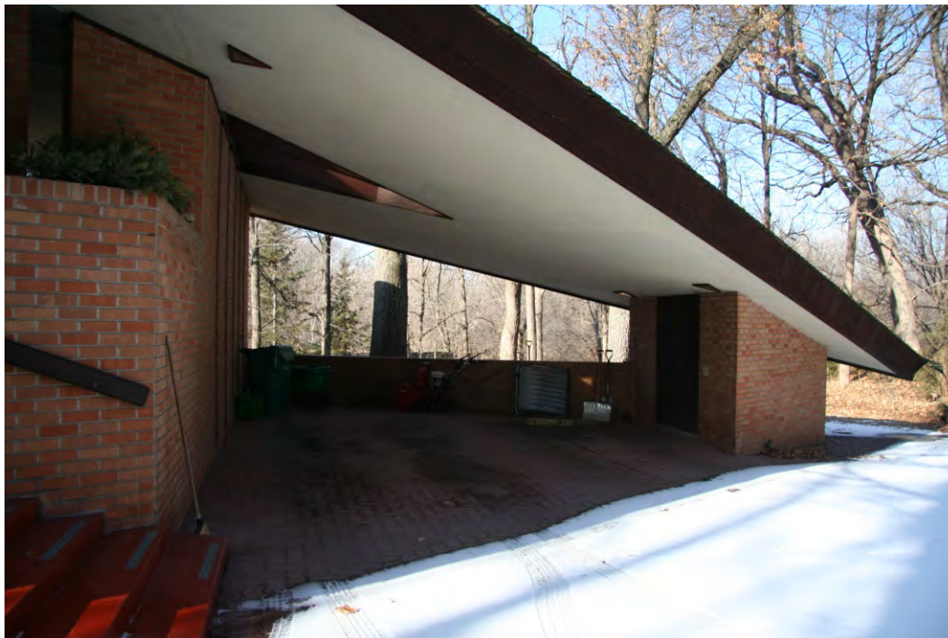
Figure 23. Overview of the carport with storage space and wall, view facing west.
