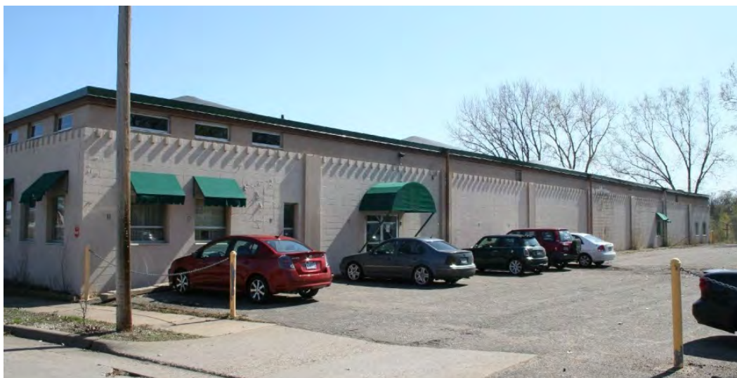
Figure 45. Southwest (side) elevation of the warehouse, view facing southeast.
