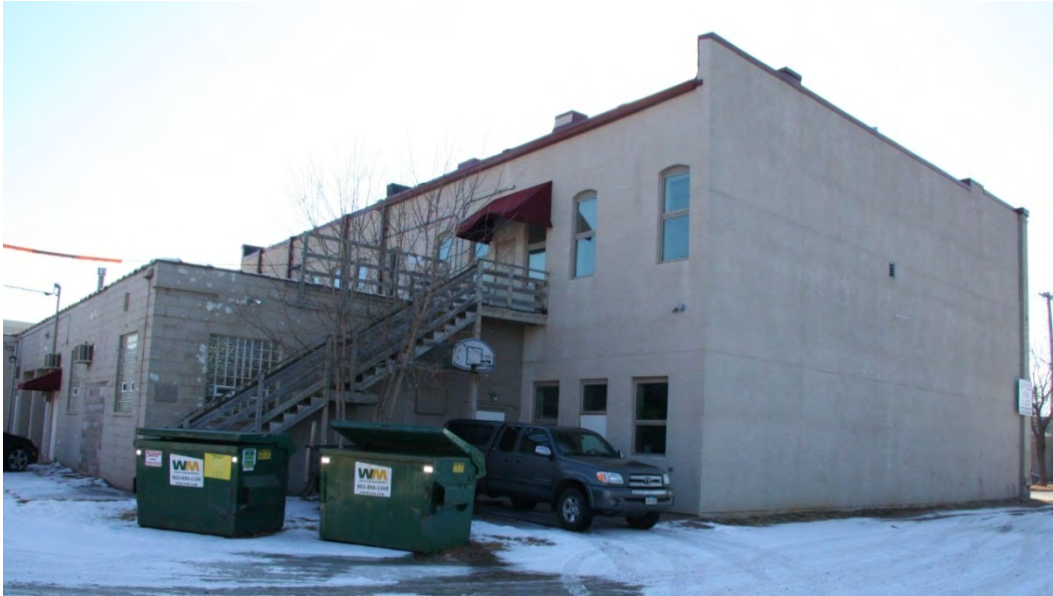
Figure 17. Walker Building, north (rear) and west (side) elevations, view facing southeast.
