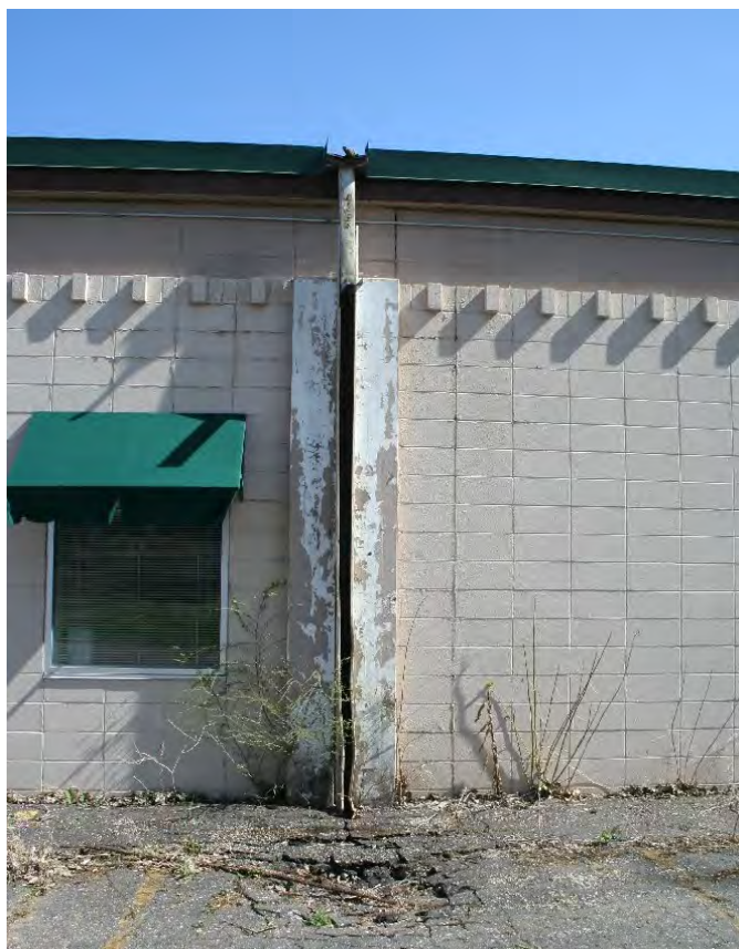
Figure 42. Concrete pilaster and aluminum downspout on southwest (side) elevation of the warehouse, view facing east.
