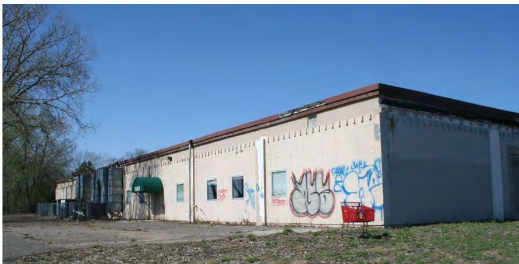
Figure 46. Southeast (rear) elevation of the warehouse, view facing northwest.
