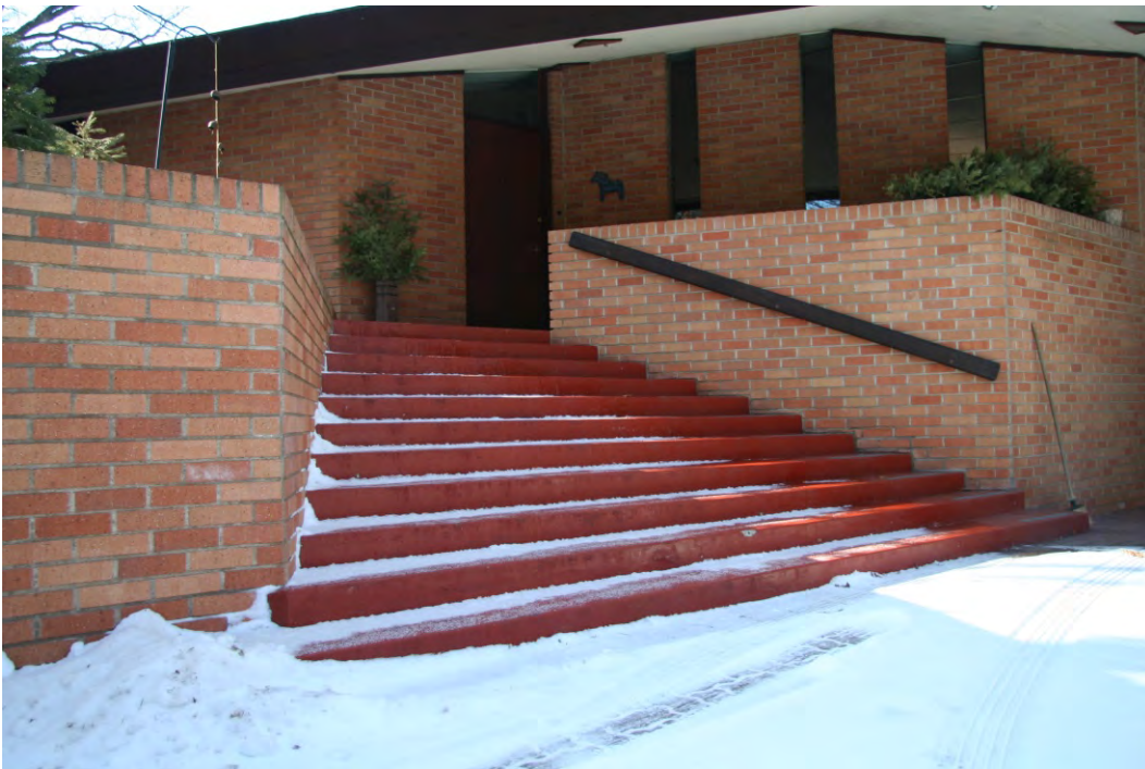
Figure 25. Entryway and stairs, view facing south.
