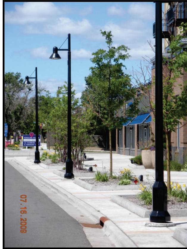
New sidewalks & lighting
