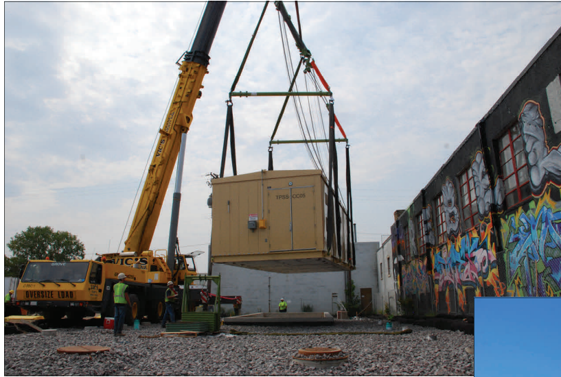
The first of 14 traction power substations was installed in late August near Raymond and University avenues.
