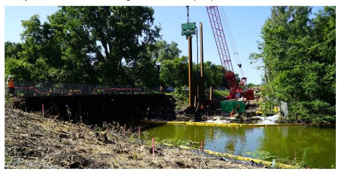
Crews work to install shoring for bridge construction at the Cedar Lake Channel. The base bridge structure will start to take shape over the next month as this and pier work progress. This area will be a focus of activity to complete this work quickly to minimize the overall impact to recreational channel water users and the surrounding community.
