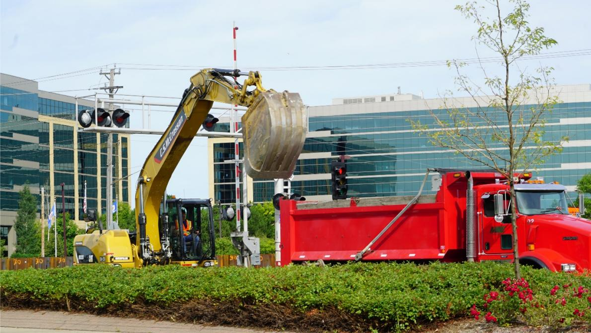
Sheet piles for the LRT bridge over Excelsior can be seen behind the excavator, as crew perform earthwork in preparation for a full closure of Excelsior.
