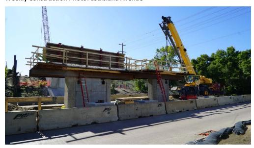
Crews constructing center bridge piers for the spans over Louisiana Avenue. Freight rail, light rail and the regional trail will all be on bridge structure over the roadway, much like today. Crews will be shifting lane closures to continue work on the bridge abutments.
