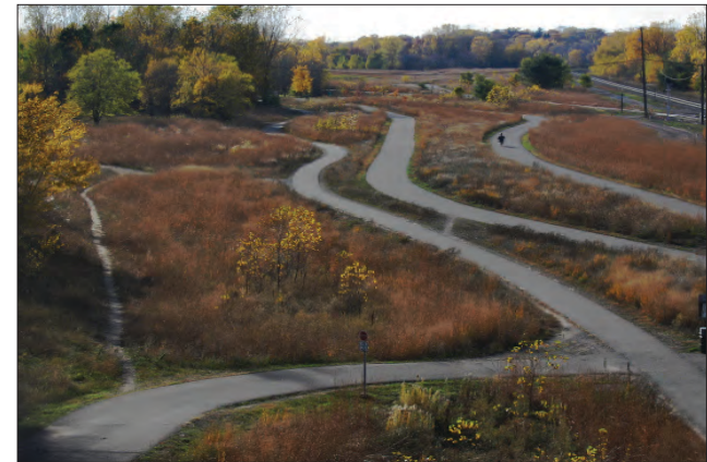
The Cedar Lake Bike Trail is a multi-use paved trail stretching nearly five miles, from Hopkins to downtown Minneapolis.
