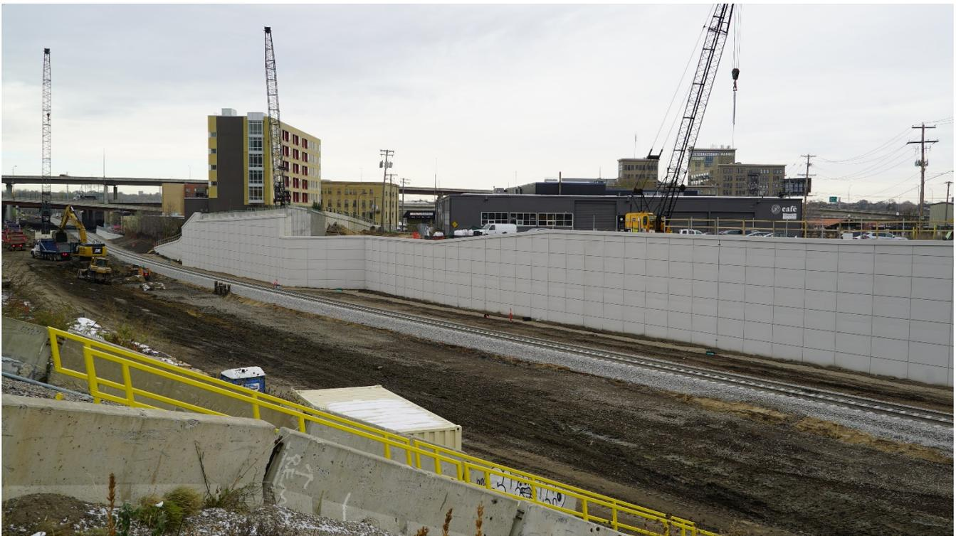
The area around Glenwood Avenue has transformed over the last year as crews built retaining walls to allow BNSF tracks to shift and make room for LRT and trail infrastructure. The new BNSF tracks can be seen in the
