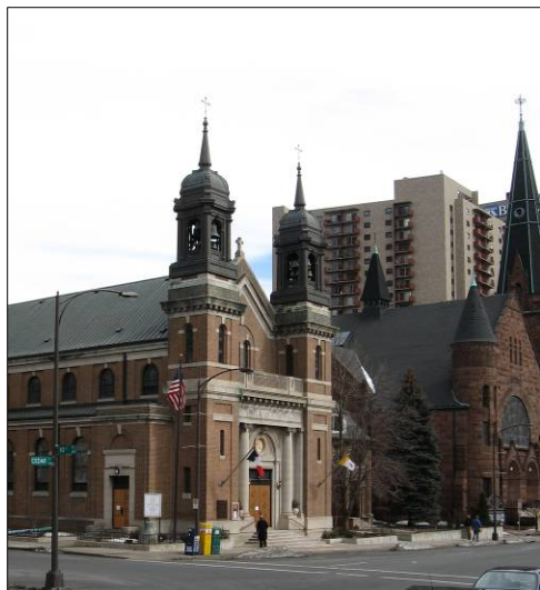
Churches in downtown St. Paul are a significant part of the visual character of Cedar Street, and are important historic landmarks. The SDEIS assesses the potential impact of the changes to the AA/DEIS LPA on these resources.
