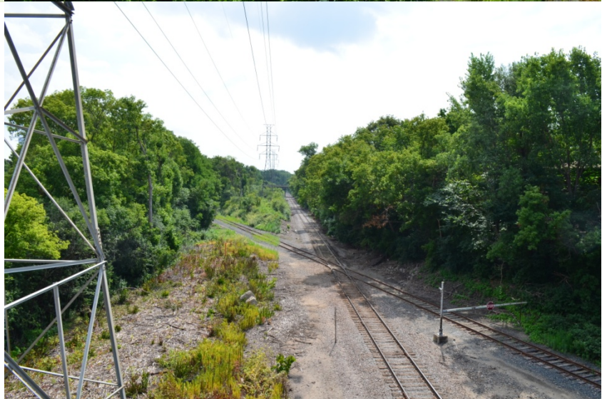
27 HE-MPC-16389 Osseo Branch, StPM&M RR Historic District (E) Minneapolis
