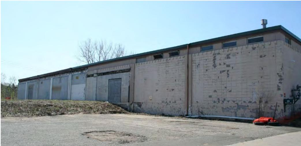
*Figure 41. Northeast (side) elevation of the warehouse showing the original wall and docking bay, downspout, and foundation, view facing south.*
