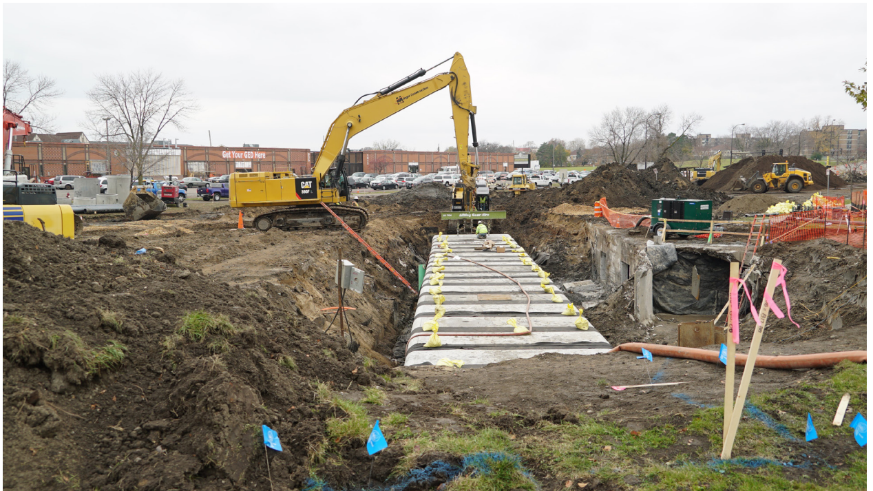
Crews install new Bassett Creek storm water tunnel starting on Oct. 30
