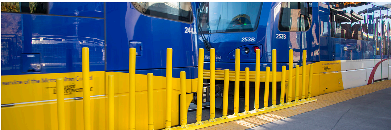
Left: Stations include safety features such as between car bollards and tactile warning strips
