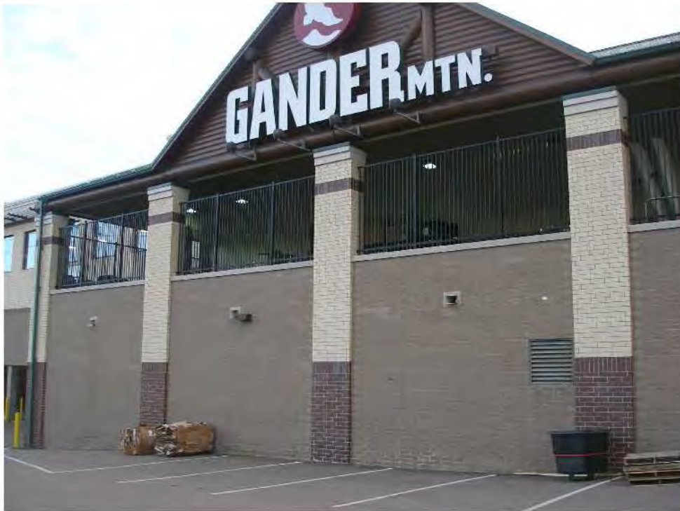
LOOKING SOUTH (THE NORTH SIDE OF THE BUILDING)
