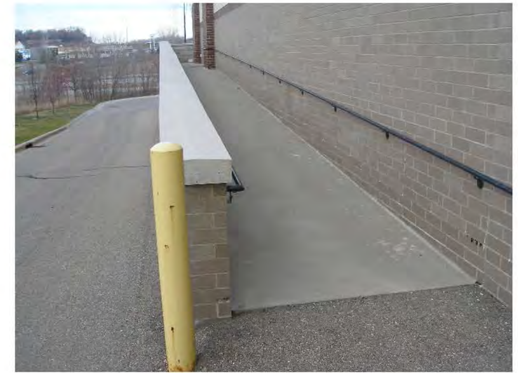
LOOKING NORTH (WEST SIDE OF THE BUILDING)
