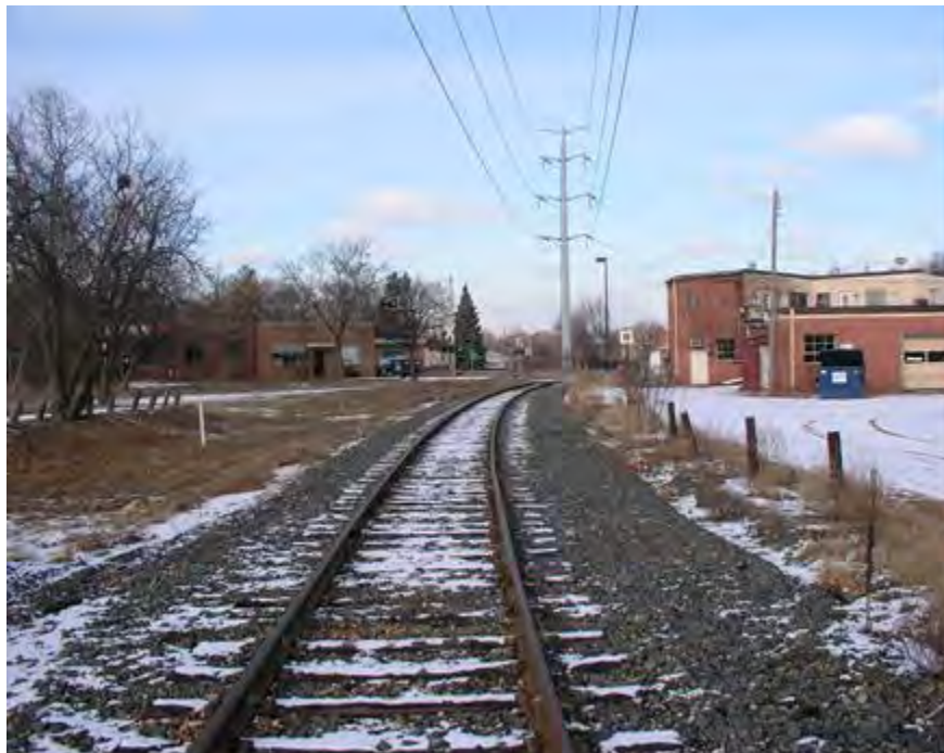
Figure #2- Locomotive Engineer's viewpoint when approaching the Walker Street crossing from the North. This is the same distance and opposite direction as from Library Lane from the North. 243 ft. of visibility.
