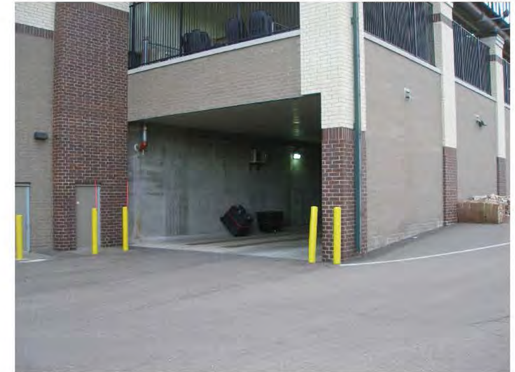
LOOKING SOUTHWEST (THE NORTH SIDE OF THE BUILDING)
