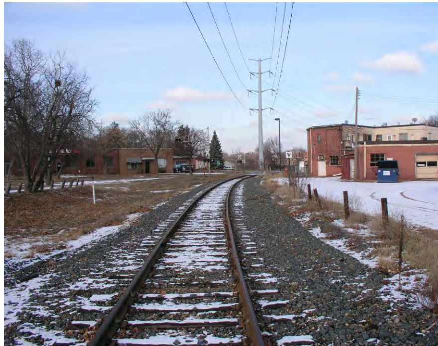
Figure #4 - Locomotive Engineer's viewpoint when approaching the Library Lane Crossing from the South. 243 ft. of visibility.
