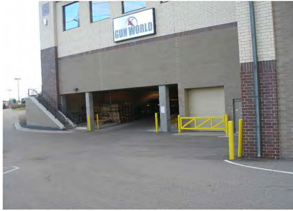
LOOKING SOUTH (THE NORTH SIDE OF THE BUILDING)
