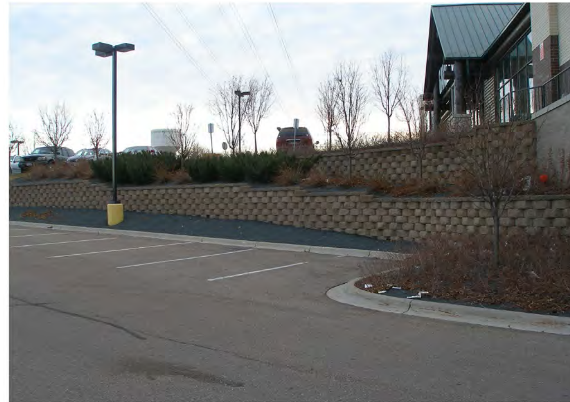
LOOKING SOUTH AT RETAINING WALL
