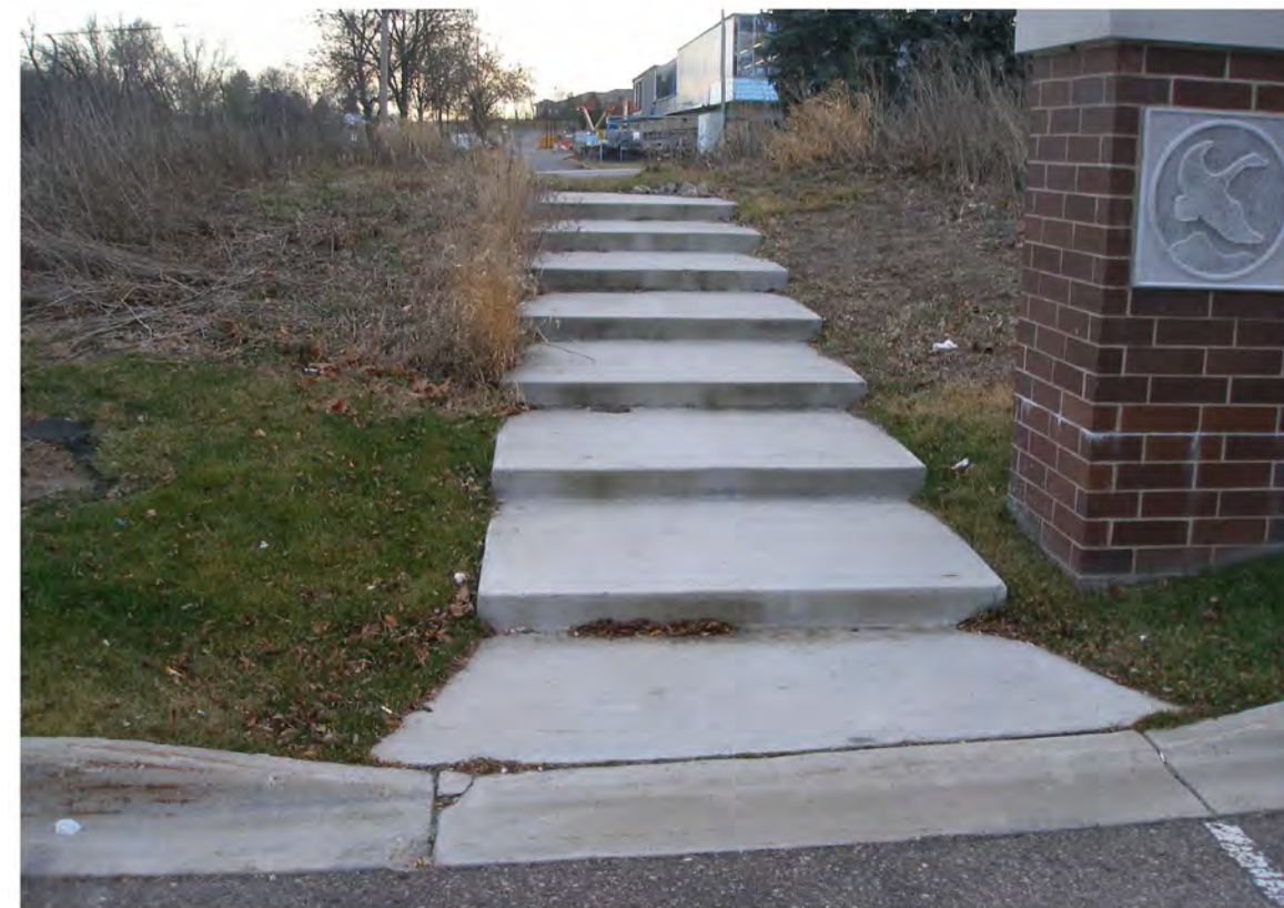
LOOKING SOUTH AT PEDESTRIAN STAIRS/WALKWAY (ON THE SOUTHSIDE OF GANDER MOUNTAIN)
