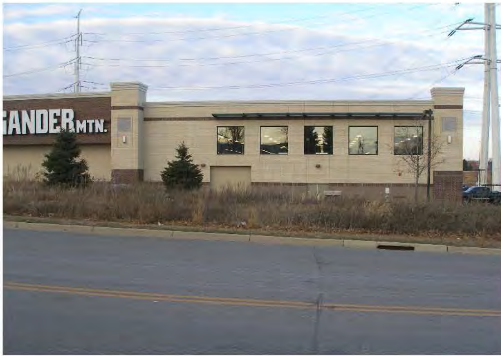
LOOKING NORTH (SOUTH SIDE OF BUILDING)
