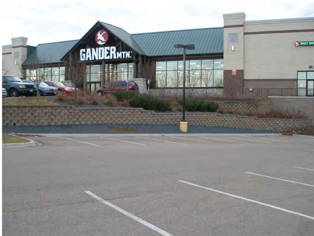
LOOKING WEST AT RETAINING WALL
