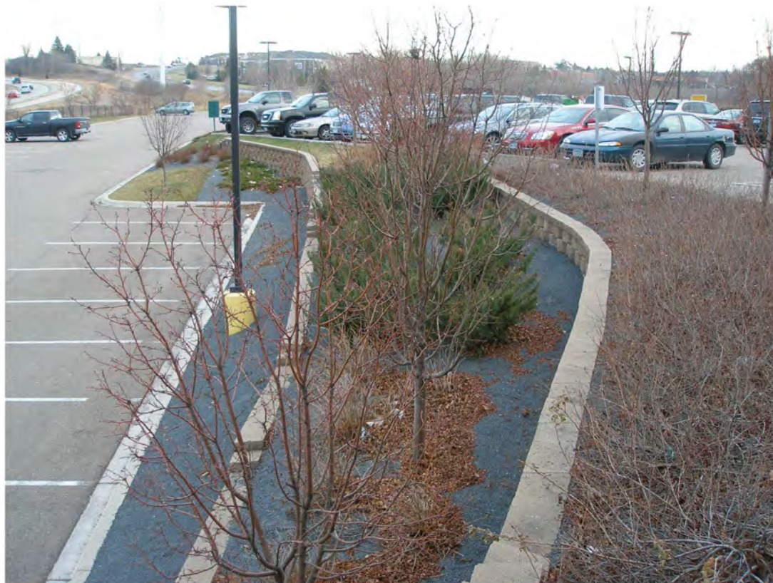
LOOKING EAST AT RETAINING WALL
