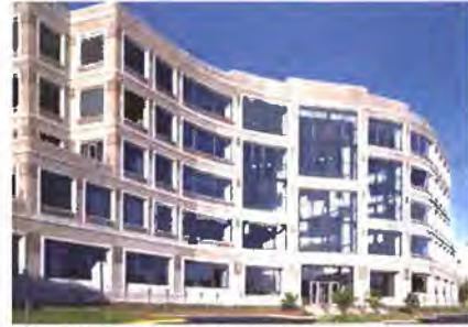
One Southwest Crossing
