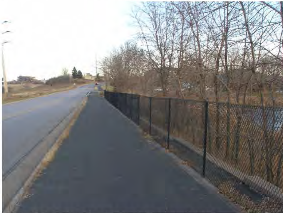
LOOKING EAST AT TRAIL ALONG TECHNOLOGY DRIVE
