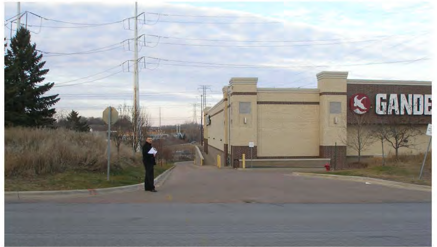
LOOKING NORTH AT THE WEST TRUCK ENTRANCE TO GANDER MOUNTAIN
