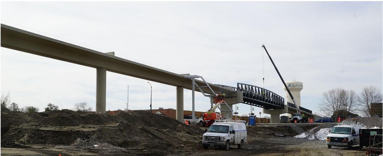
Crews can be seen working on the Beltline Boulevard pedestrian bridge in St. Louis Park, installing the metal stair towers as an alternative option for accessing the pedestrian bridge.
