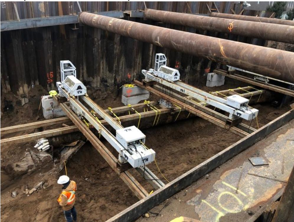
Crews have completed a move of the CenturyLink duct bank on Glenwood Avenue in Minneapolis. Moving this major utility allows crews to begin work on the west abutment of the Glenwood Bridge in 2020. Crews have begun to backfill the trench, pictured above.
