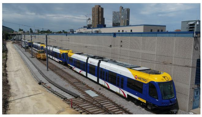
To accommodate the new light rail vehicles (LRVs) needed for the Southwest Project, expansion of the Franklin Operations and Maintenance Facility is underway. Four LRVs are pictured next to new tracks on the west side of the facility. New Overhead Catenary System (the poles and wires) were also constructed.
