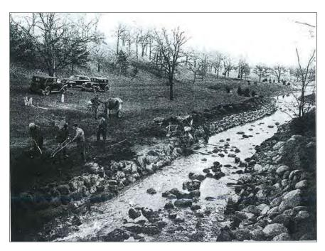
Figure 9. Federal relief workers placing riprap along Bassett Creek (MBPC 1941:33).
