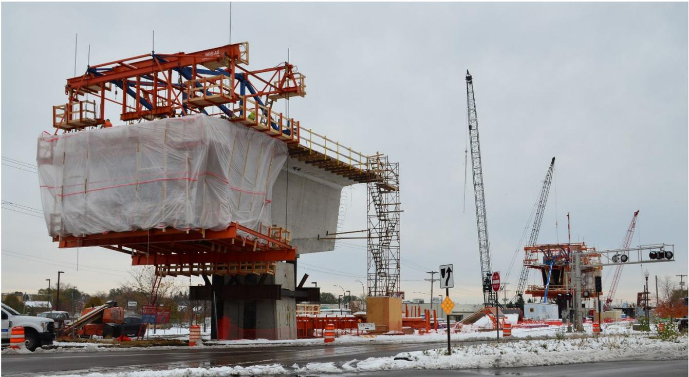
The LRT bridge spans continue to take shape at Excelsior Boulevard in Hopkins. To construct the bridge, crews are using a system called a form-traveler to build the spans between the piers. Instead of setting beams, the bridge structure is formed a section at a time. The bridge structure is called a post-tensioned box girder bridge,
