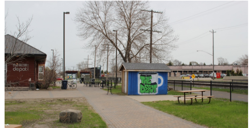
Hopkins Depot: Before
