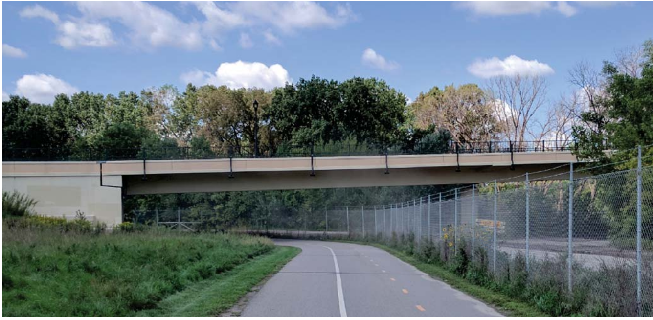
The light color bridge pops out of the landscaping. The girder creates shadow helping part of the bridge blend into the background.
