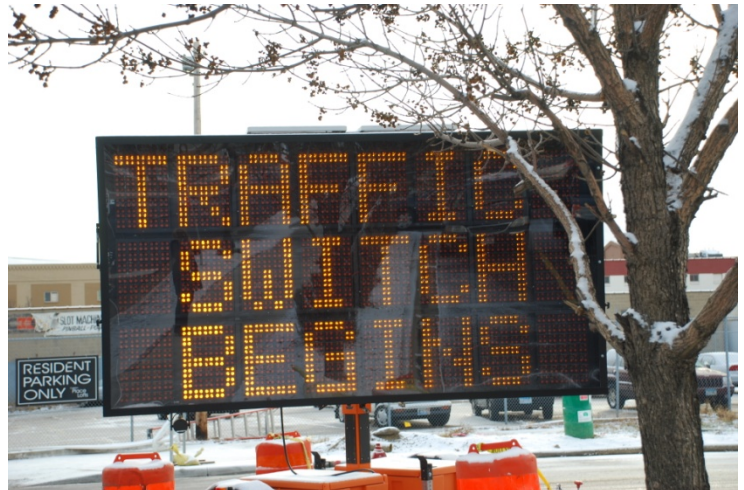
VMS used to alert drivers to the traffic switch on University Avenue
